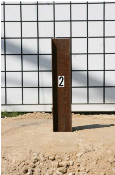
Figure D3. Steel posts over underground structure with 48-inch concrete footing before test 405160-12 P2.
