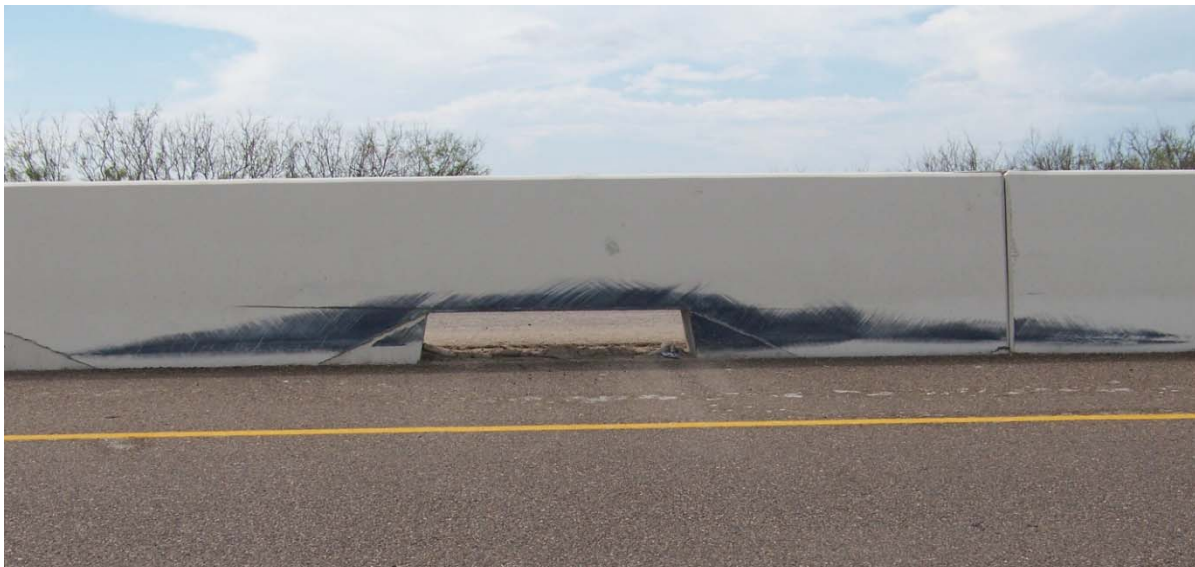
Figure 4 – Vehicle Impact at 12-inch High Opening in TXDOT Wildlife Crossing Barrier.
