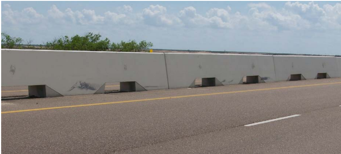
Figure 3 – TXDOT Single Slope Concrete Barrier (Wildlife Crossing) SSCB.
