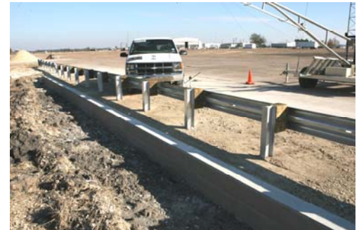
W-Beam Guardrail on Box Culvert
