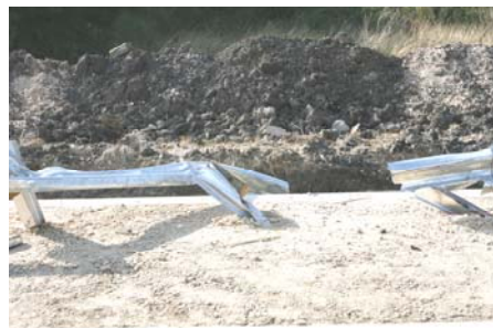
Barrier after Test
