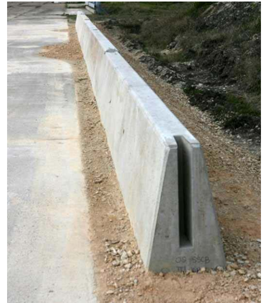
Single-Slope Barrier in Front of 1.5H:1V Slope
