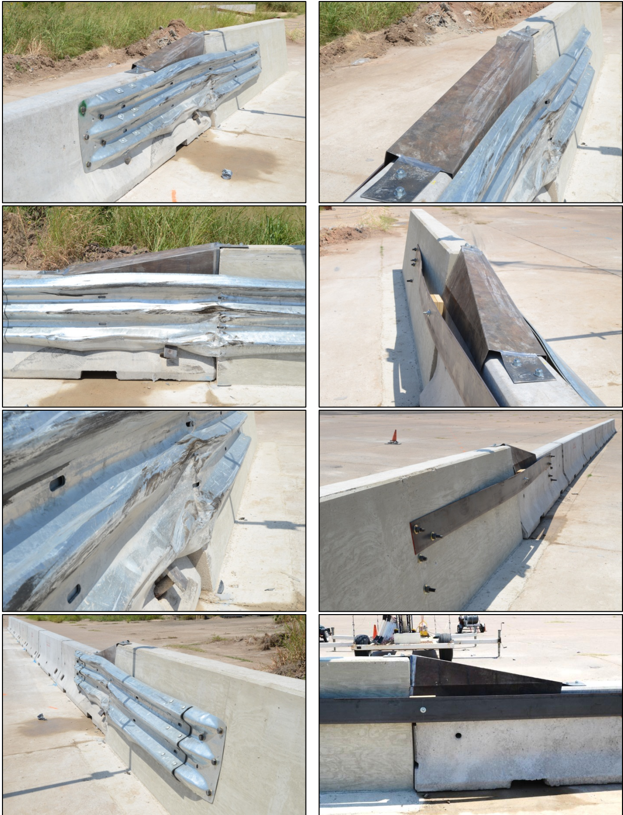
Figure 6.4. Installation after test 405160-34-1.
