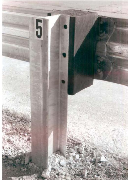
**(a) Strong post with Steel Post Guardrail (G4(1S)) (TTI 400001-MPT1) (21).**
