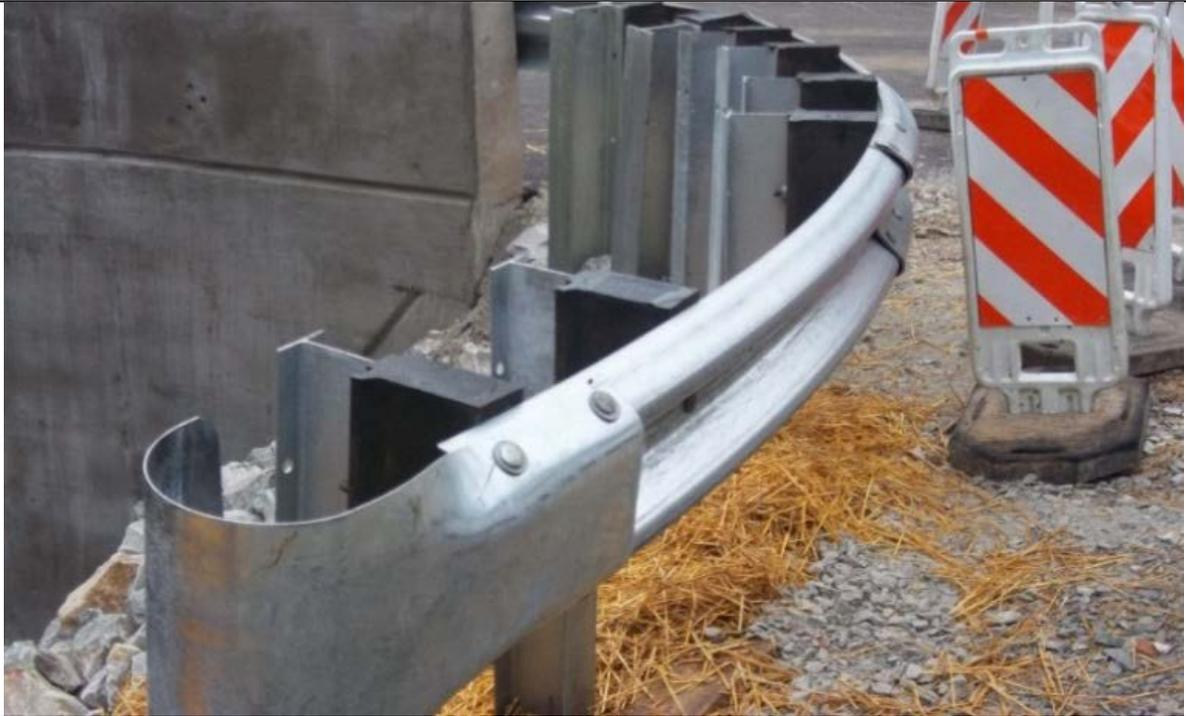
(b) Short Radius Guardrail Example from Pennsylvania DOT
