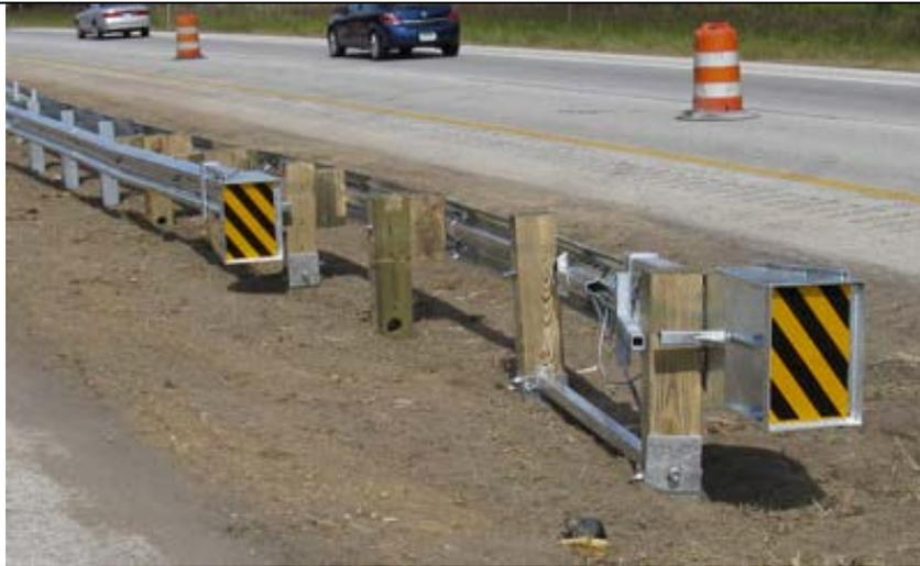
**FLEAT-MT** – a median terminal commonly used in wide medians. Depending on the severity of the impact, vehicle can be stopped before reaching the second impact head. Meets TL-3 test criteria.
