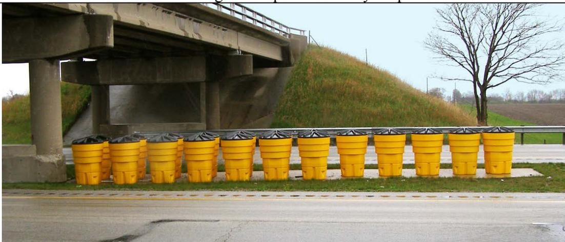
**Sand Barrels** – non-redirective, gating sand filled crash cushion. Common set up consists of 12 barrels, typically a single file of four barrels followed by 4 rows of 2 barrels in each.
