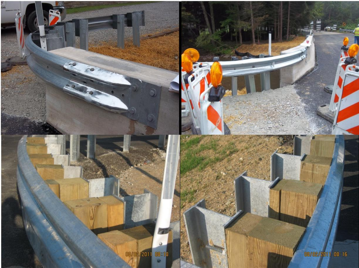
**Figure D1. Example of Short Radius Guardrail from Pennsylvania.**
