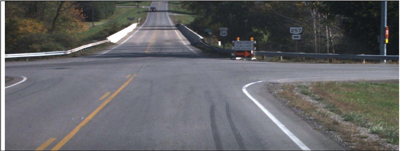
(a) Short Radius Guardrail Example from Ohio DOT
