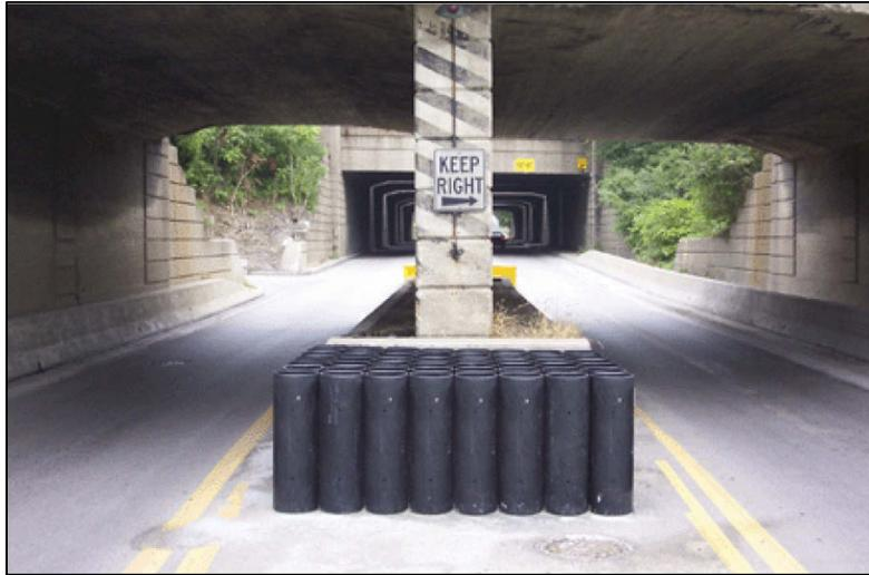
**EASI-CELL** – composed of 32, energy absorbing, reusable cylinders, can self-recover after impacts up to about 90% of its original shape without maintenance. Meets TL-1.
