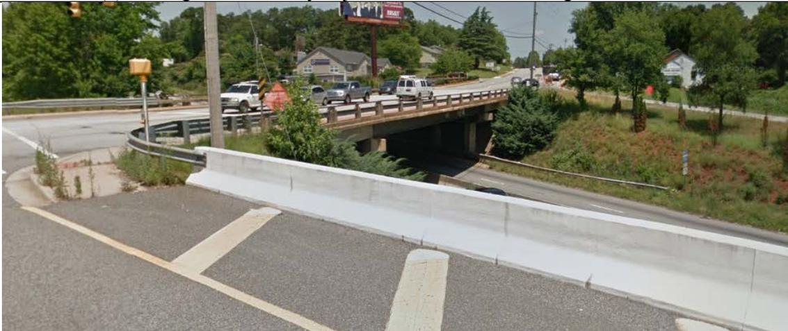
(b) “Bridge immediately adjacent to barrier on interchange ramp.” The bridge is expected to be raised 2 feet in a future project. “Barrier wall will also be adjusted and lengthened for the new fill conditions and may be extended to wrap around the radius where the existing guardrail is in place.”
