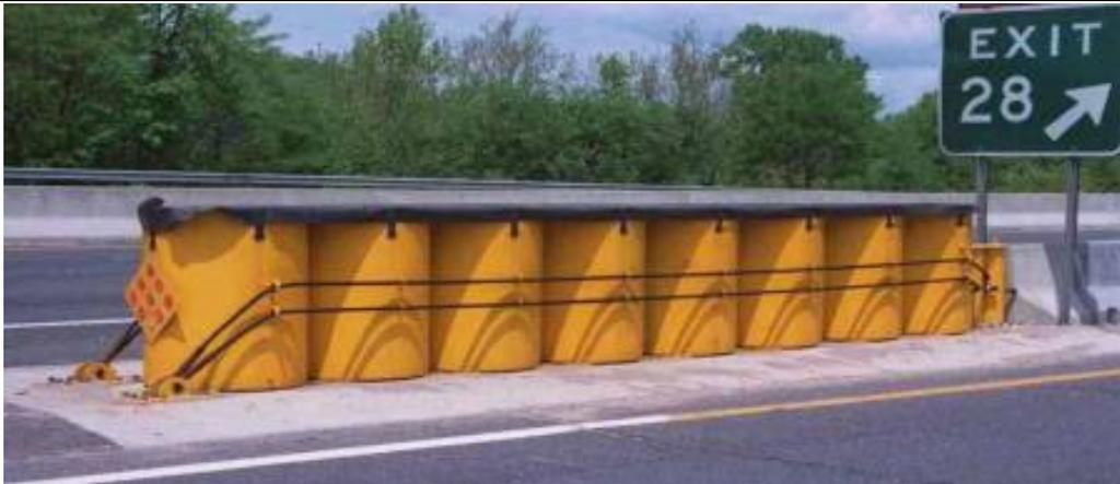
**NCIAS** (Connecticut Impact Attenuation System) – redirective, non-gating crash cushion, consists of 8 steel cylinders. Meets TL-3 test criteria.
