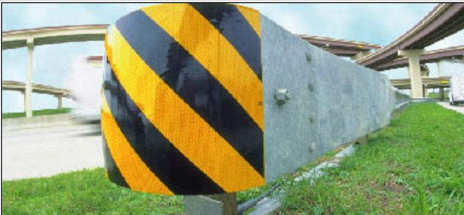
**CAT 350** (Crash Cushion Attenuating Terminal) – energy absorbing attenuator, TL-3 test criteria.
