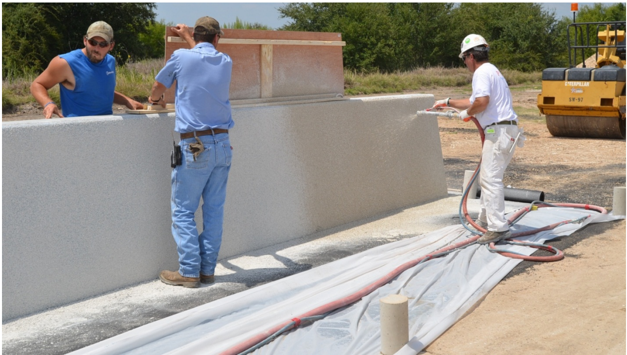
Figure 2.6. Coating Buildup of Acoustement® 40.
