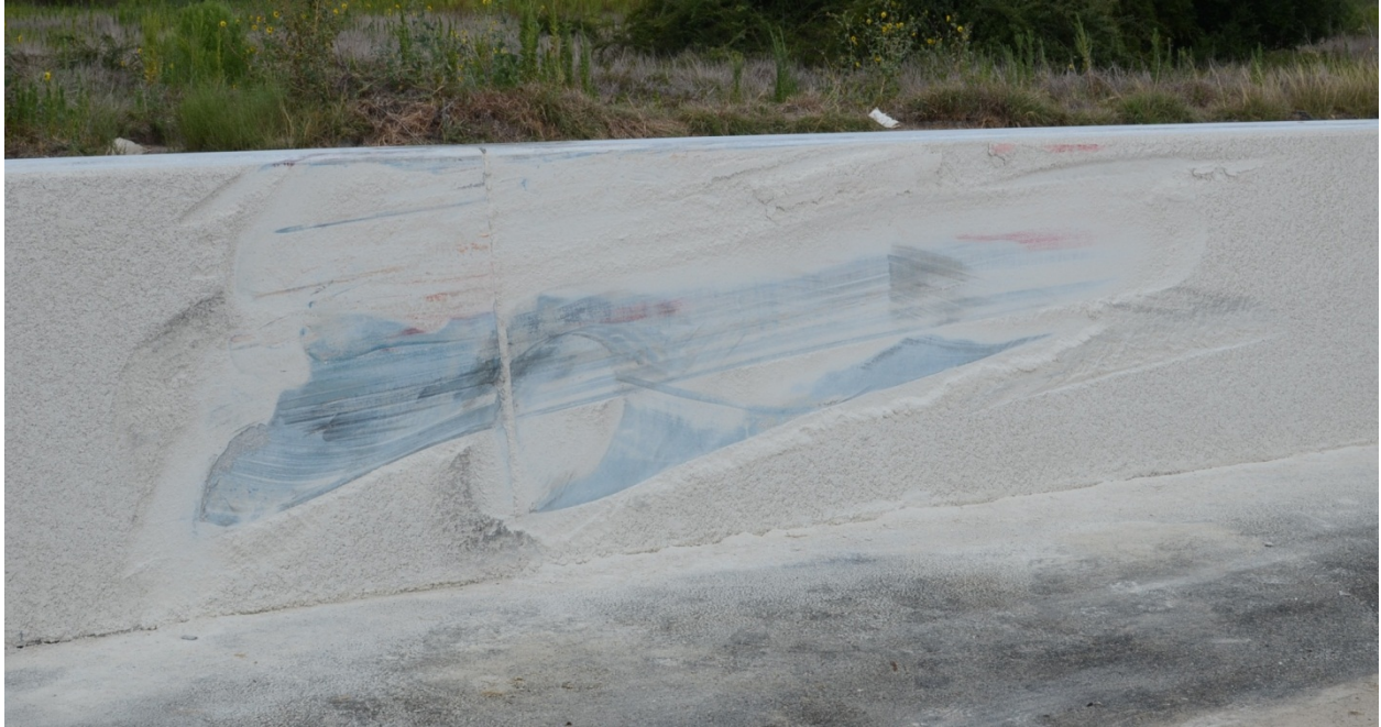
Figure 5.8. Damaged Coating after Test.
