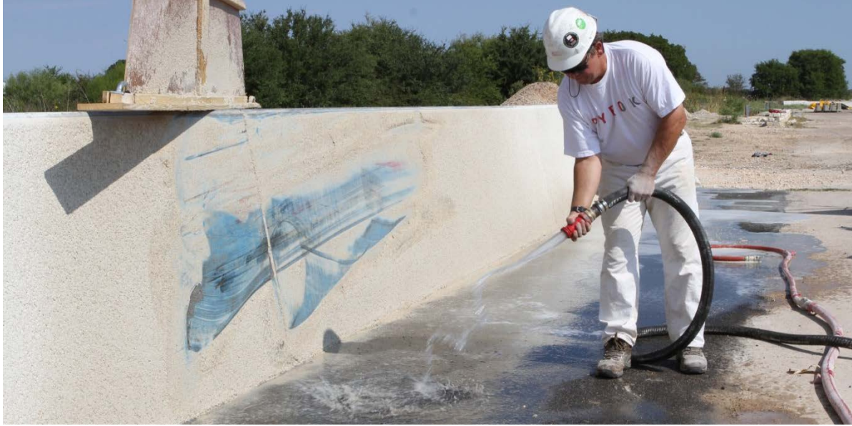
Figure 5.10. Washing Down Damaged Coating Area.
