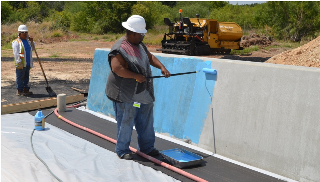
Figure 2.3. Application of Weld-Crete® Concrete Bonding Agent.
