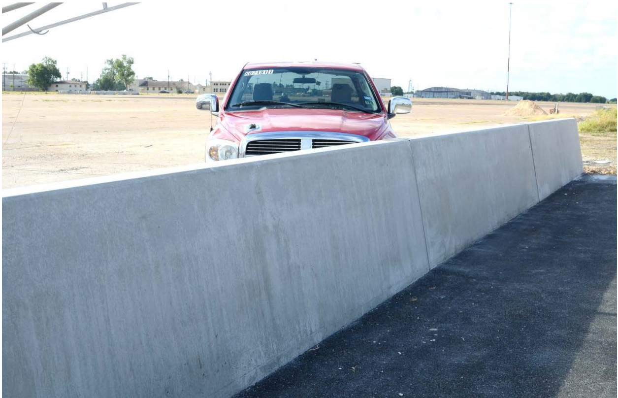
Figure 5.1. Vehicle/Installation Geometrics for Test No. 602191-1.
