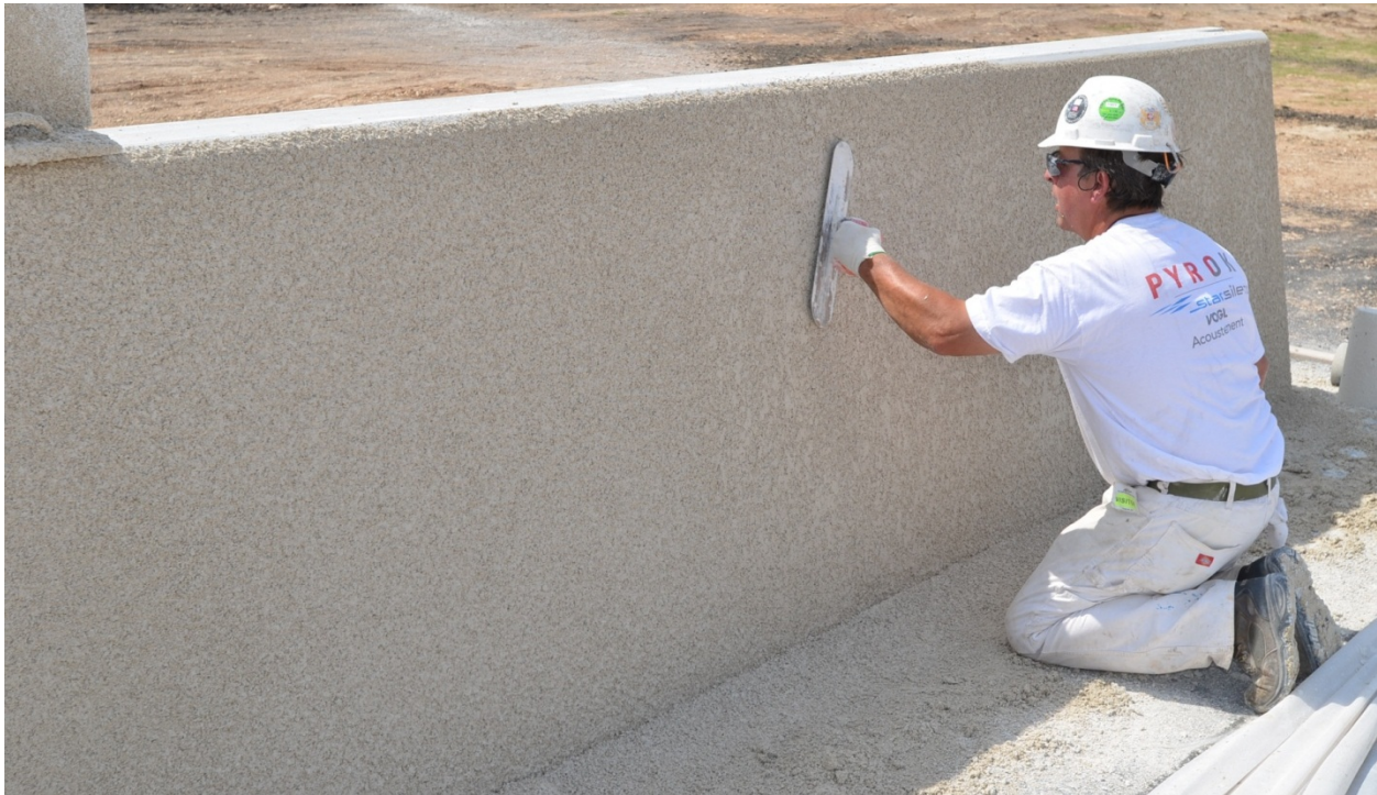
Figure 2.8. Light Hand Finishing of Acoustement® 40 coating.
