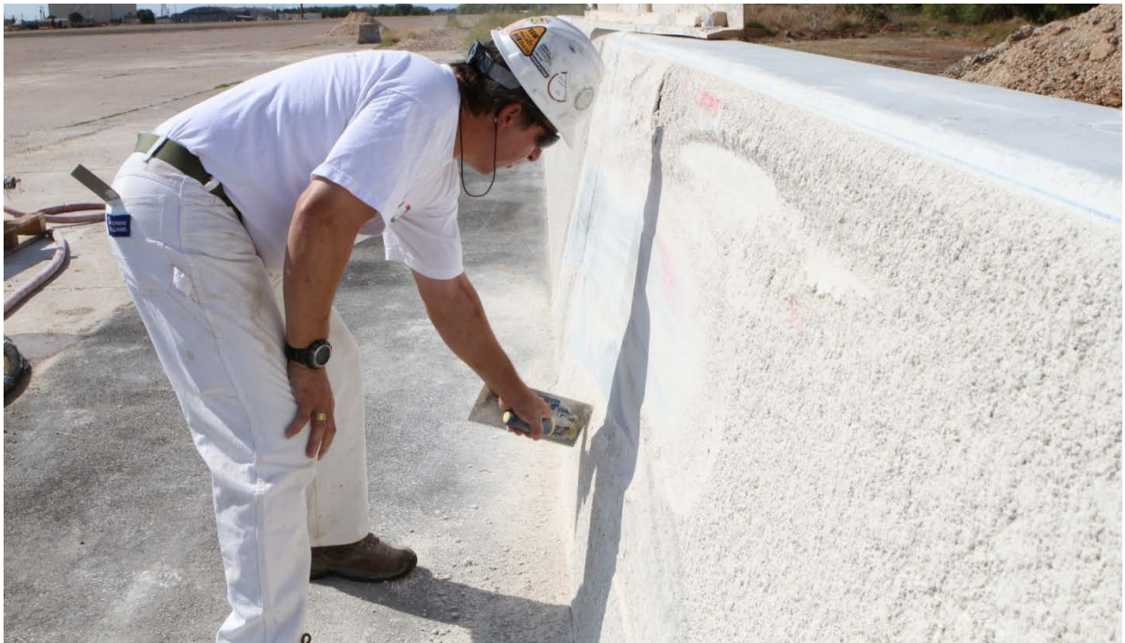
Figure 5.9. Preparing Edges of Damaged Coating for Repair.
