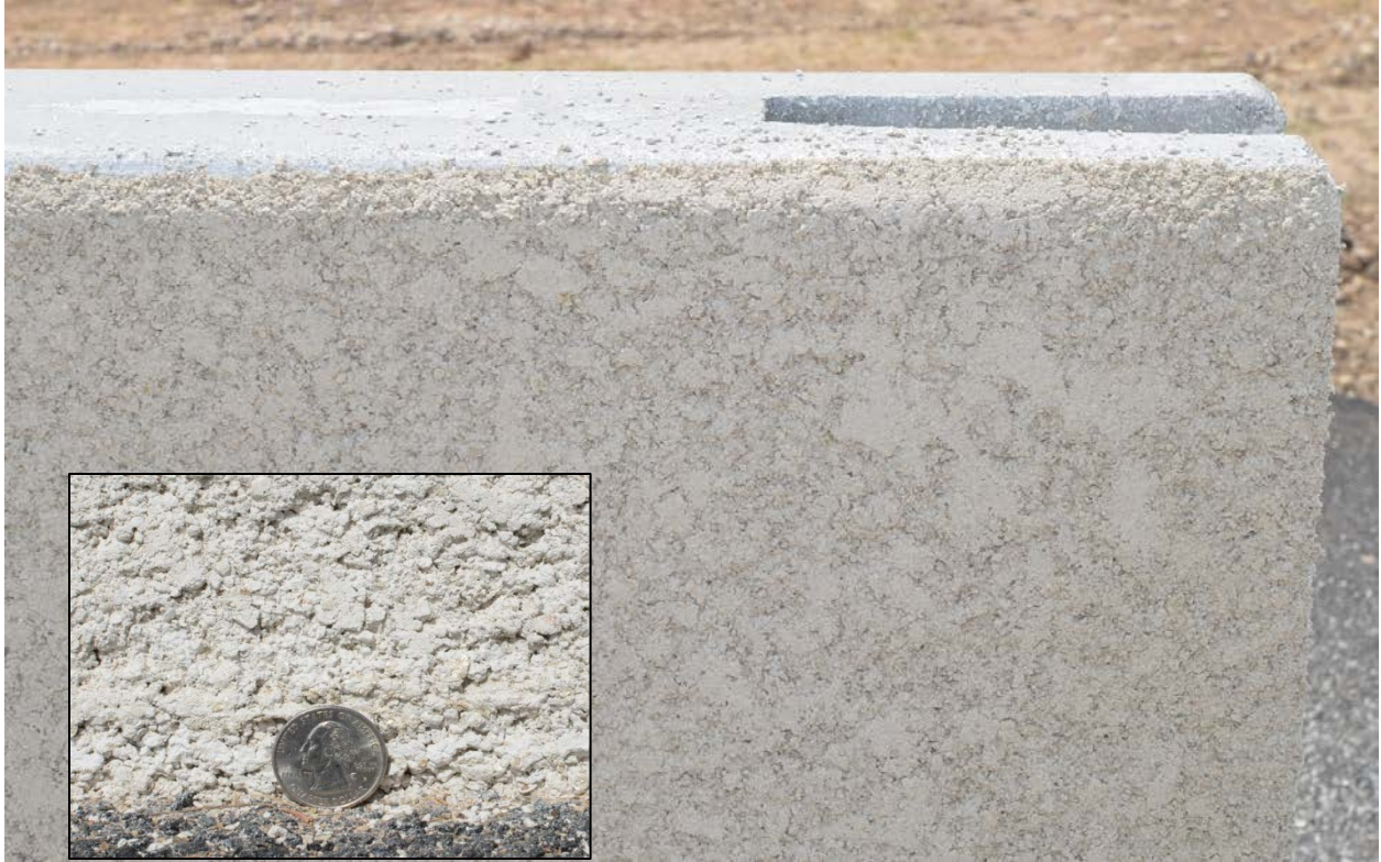
Figure 2.9. Finished Acoustement® 40 coating.
