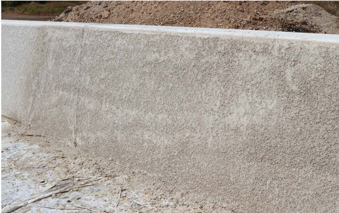
Figure 5.13. Repaired Coating.
