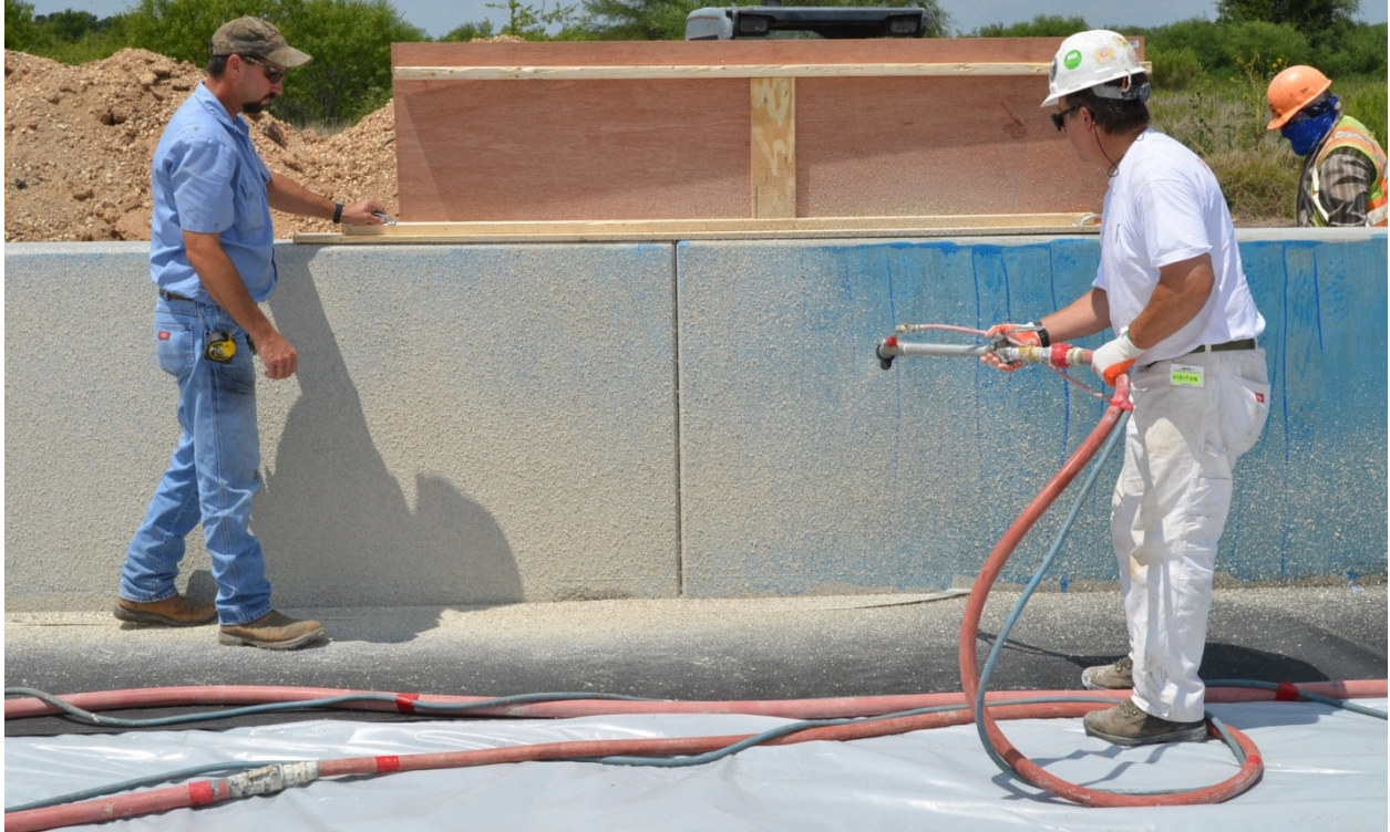
Figure 2.5. Application of First “Key” or “Flock” Coat of Acoustement® 40.
