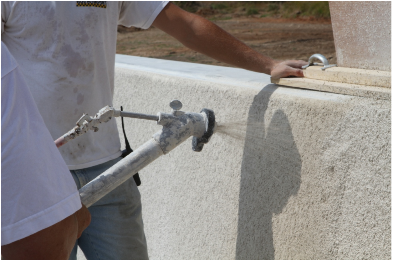
Figure 5.11. Application of Repair Coat.
