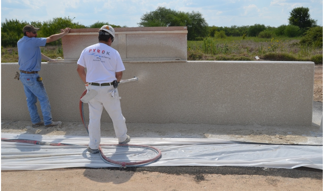
Figure 2.7. Application of Final Coat of Acoustement® 40.
