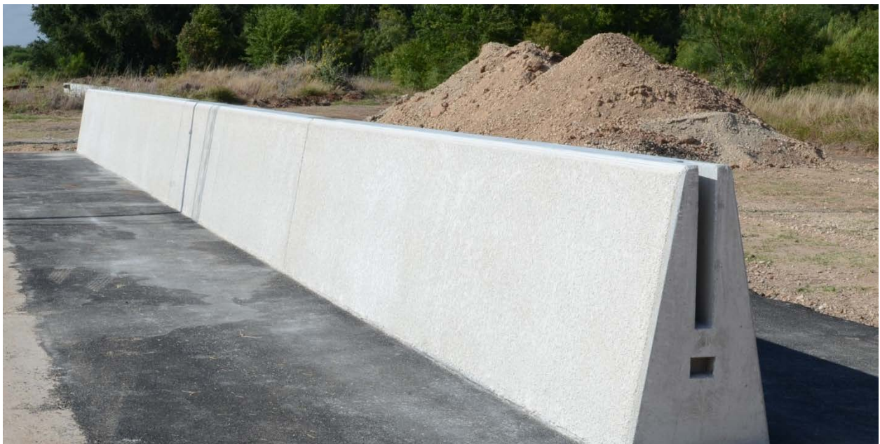
Figure 2.10. Completed test installation.
