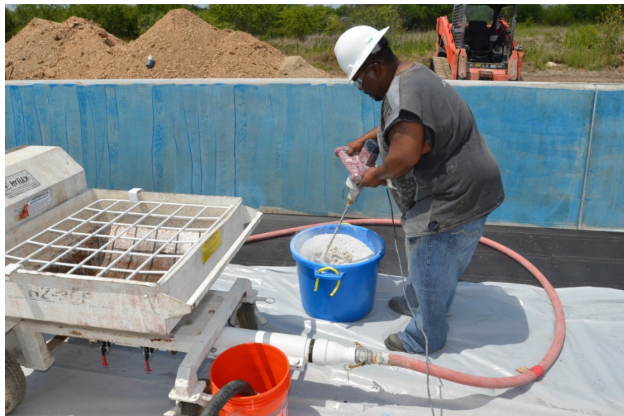
Figure 2.4. Mechanical Mixing of Acoustement® 40.
