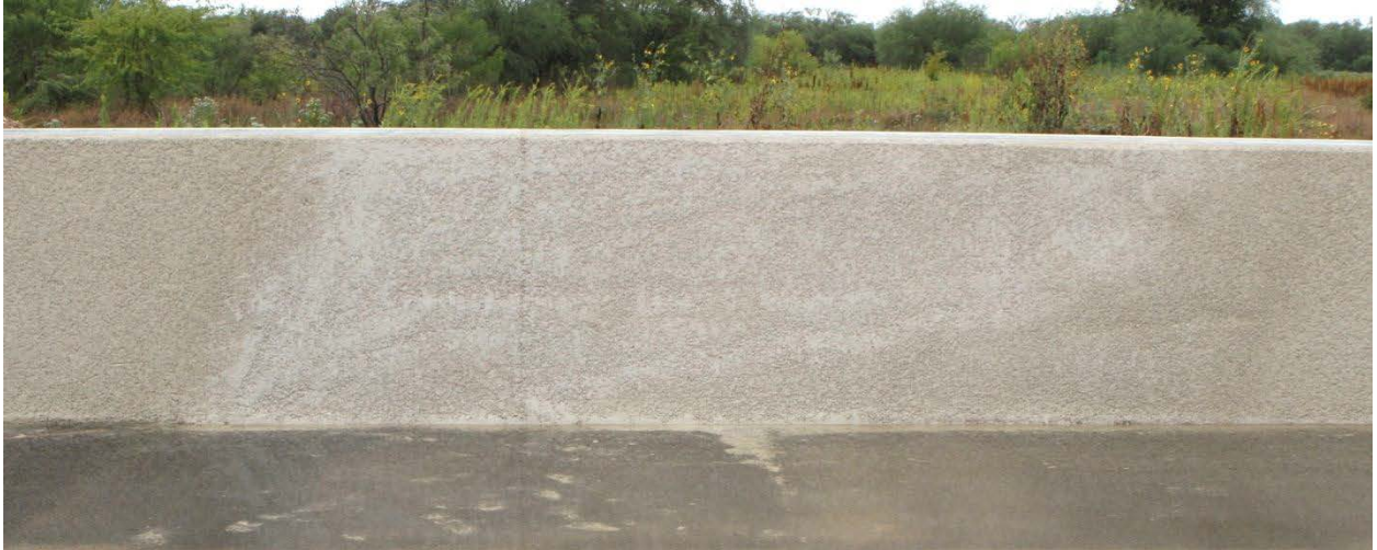
Figure 5.14. Repaired coating after rain.
