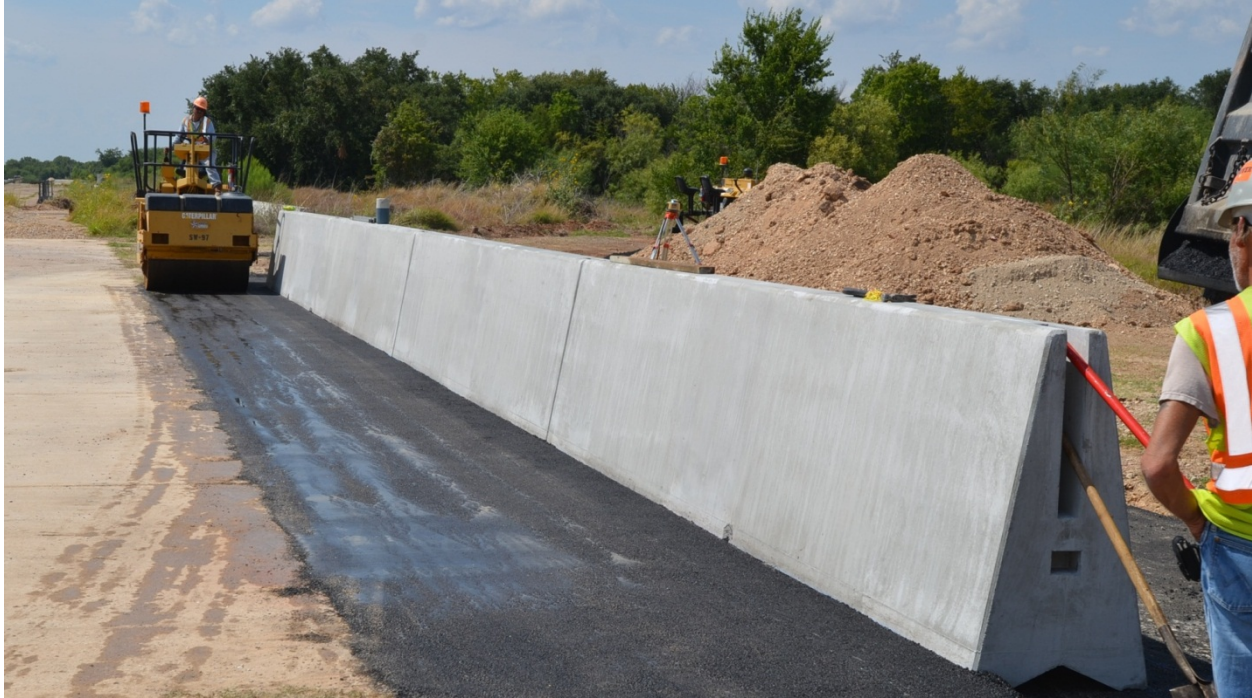
Figure 2.2. Compaction of 3-inch Asphalt Overlay/Key.
