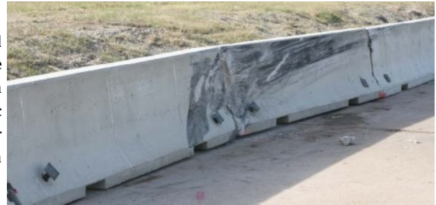
Temporary Barrier on Concrete after Crash Test
