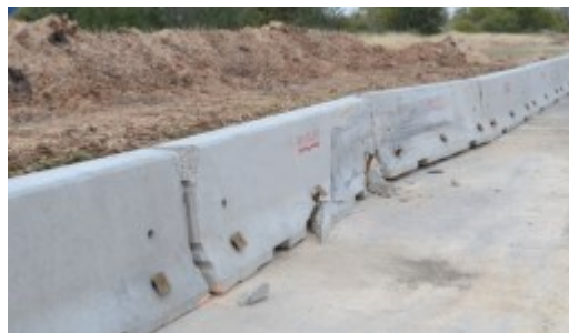
Installation after Crash Test
