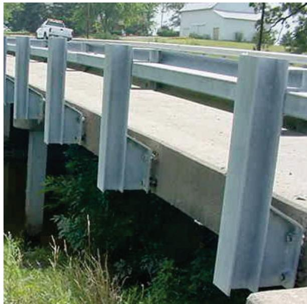
Figure 1 – Ohio Department of Transportation Side Mount Bridge Rail
