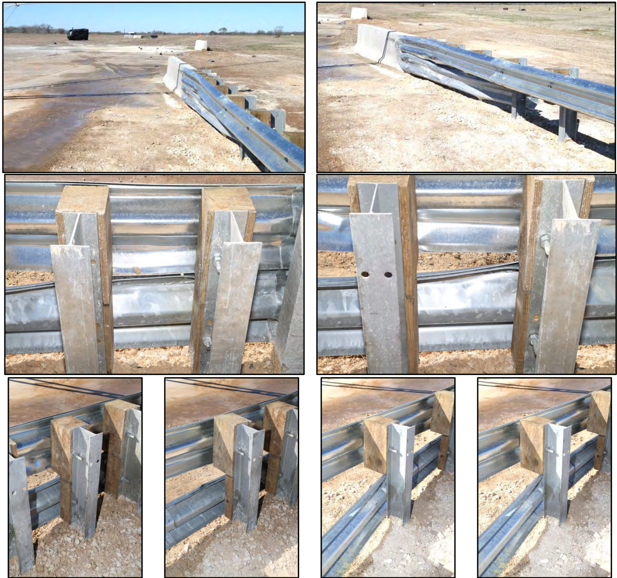
Figure 2. Stacked W-Beam Transition after Test No. 604581-1.
