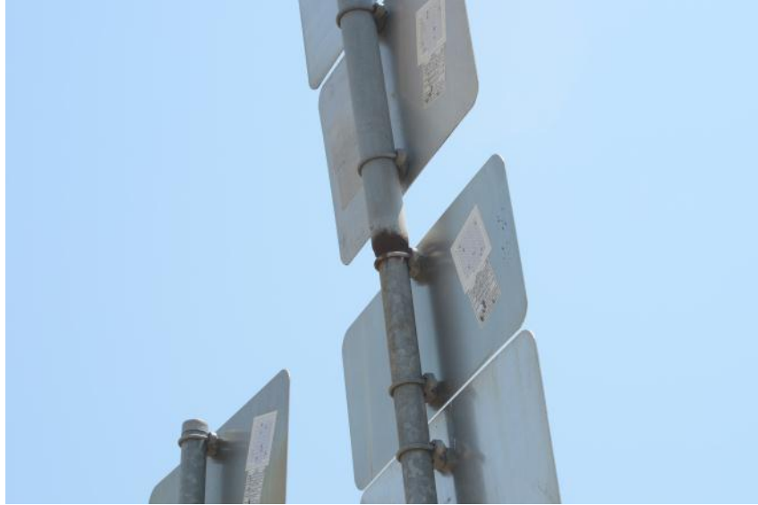
Figure 11.3. Improper Installation of U-Bracket Extension Tube.
