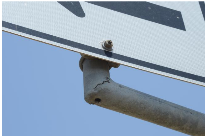
Figure 11.2. U-Bracket Weld Failure.
