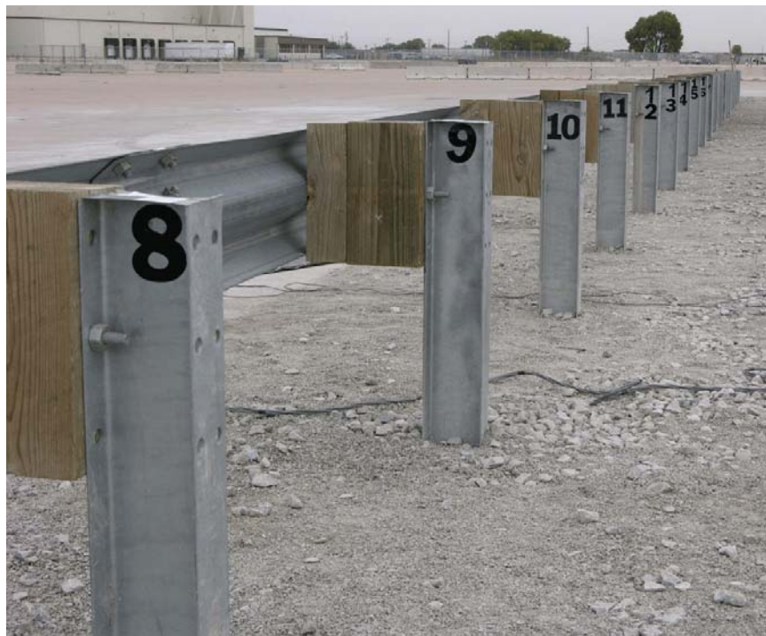
Figure 12. Midwest Guardrail System
