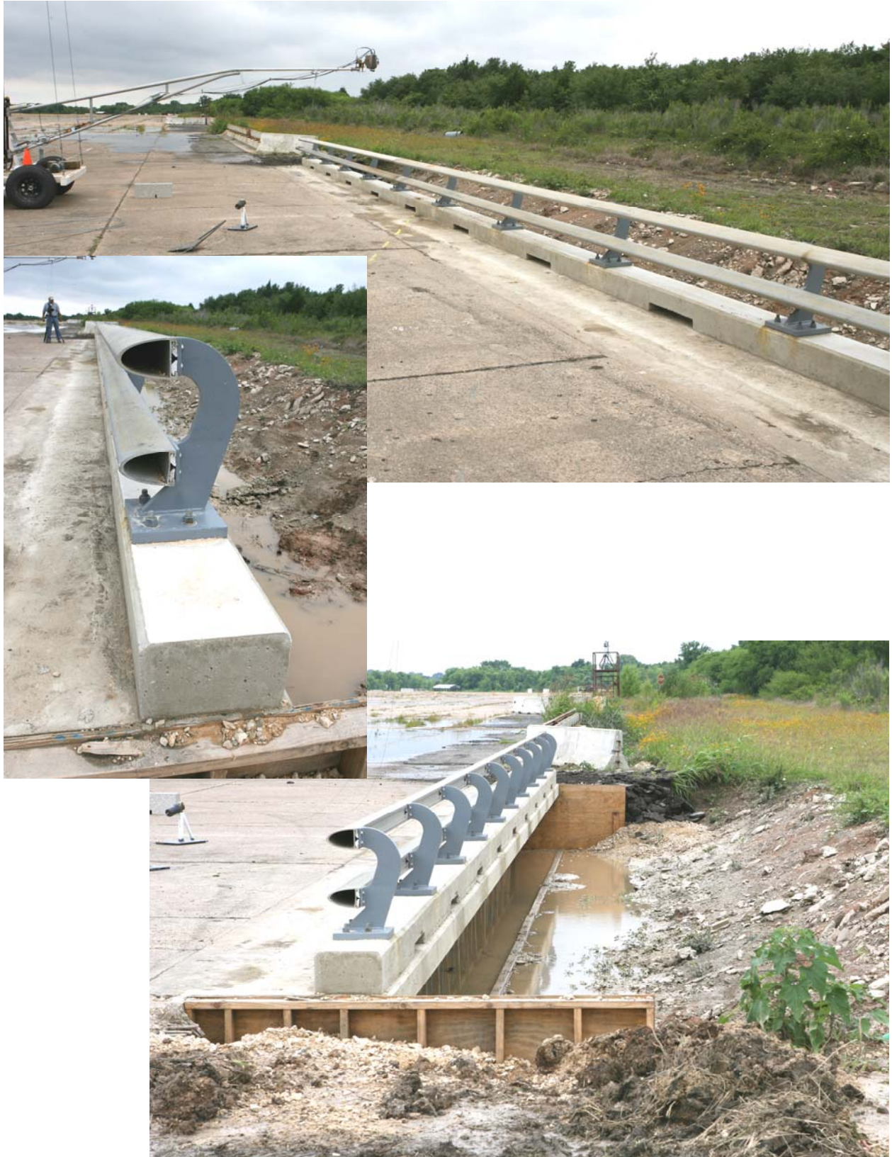
Figure 2.3. TxDOT T-1F Bridge Rail Installation Before Test 408019-1.
