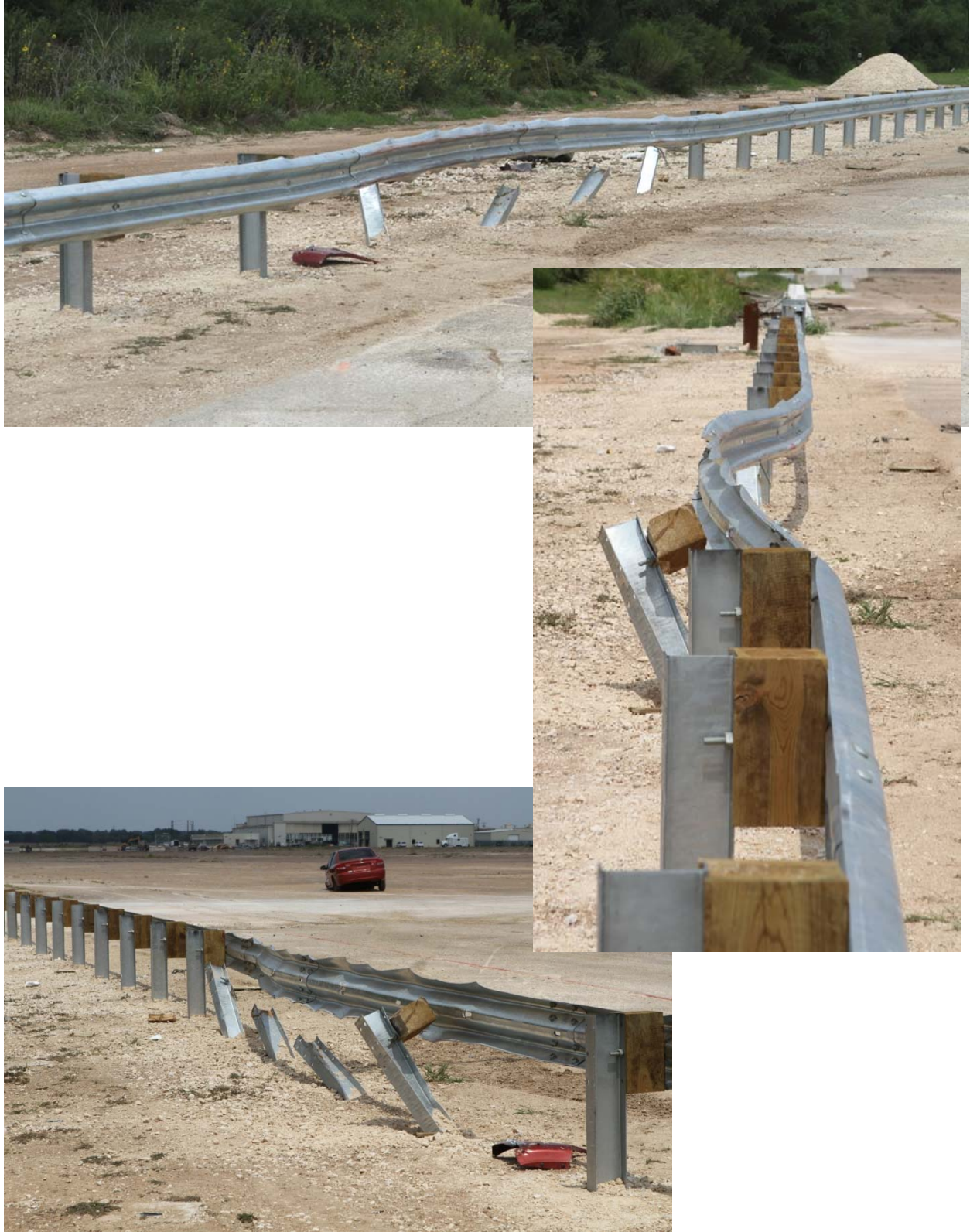
Figure 5.4. Installation after Test No. 420020-5.
