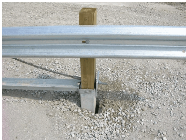
Figure 41. Downstream Anchorage Damage, Test No. MGS221-1
