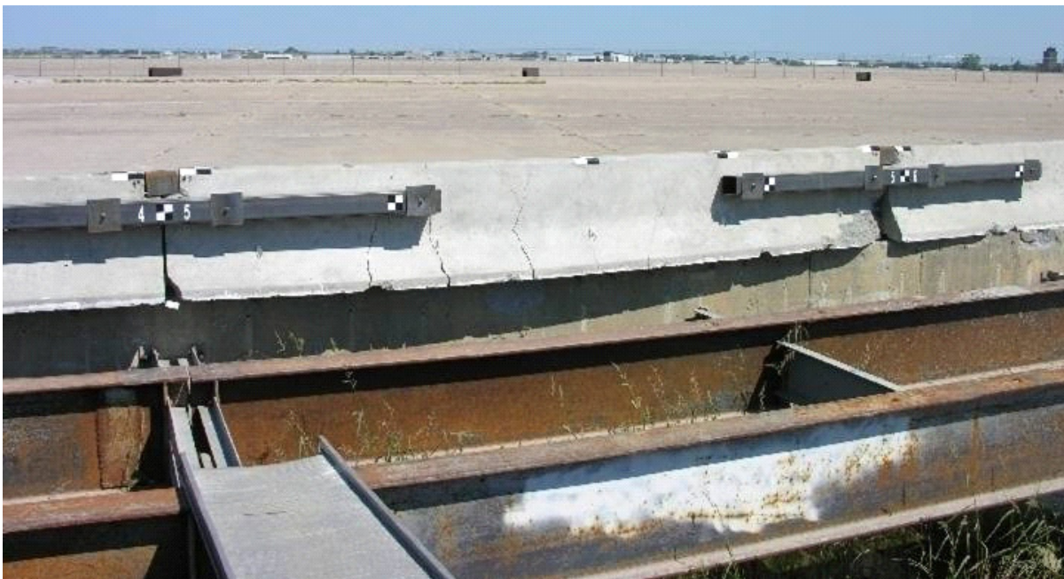
Figure 80. Box Beam Stiffened Temporary Barrier Damage, Test NYTCB-3
