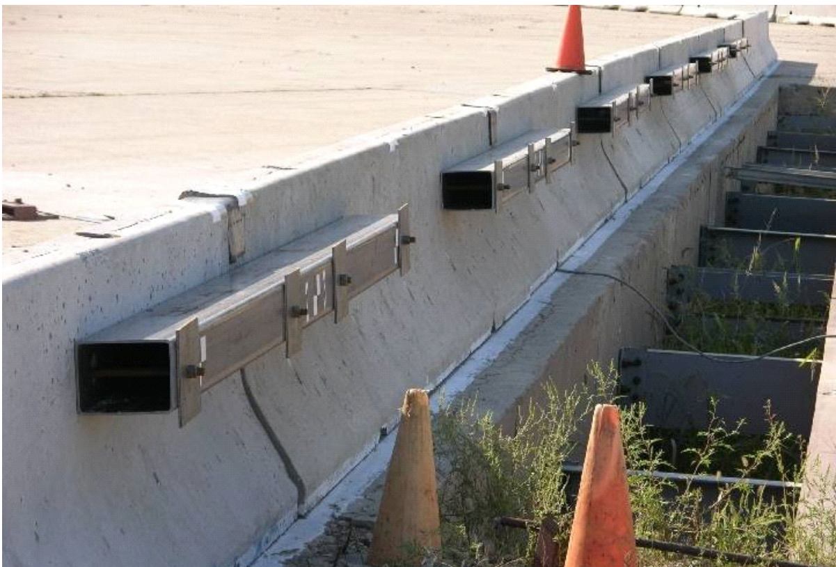
Figure 69. Box Beam Stiffeners, Test NYTCB-3
