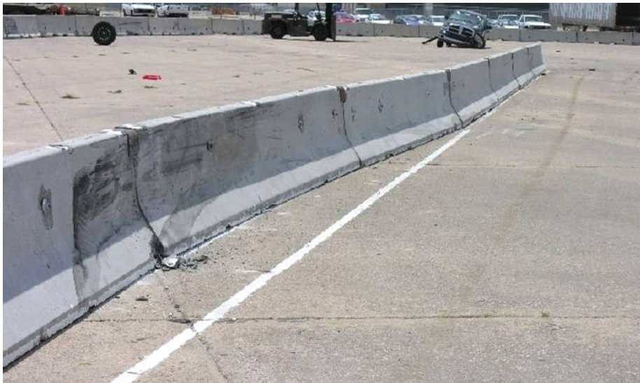
Figure 36. Vehicle Final Position and Trajectory Marks, Test NYTCB-1
