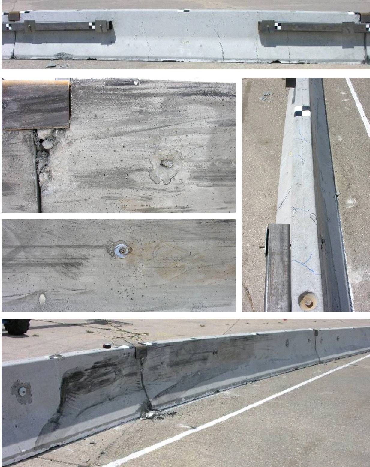
Figure 39. Barrier No. 5 Damage, Test NYTCB-1
