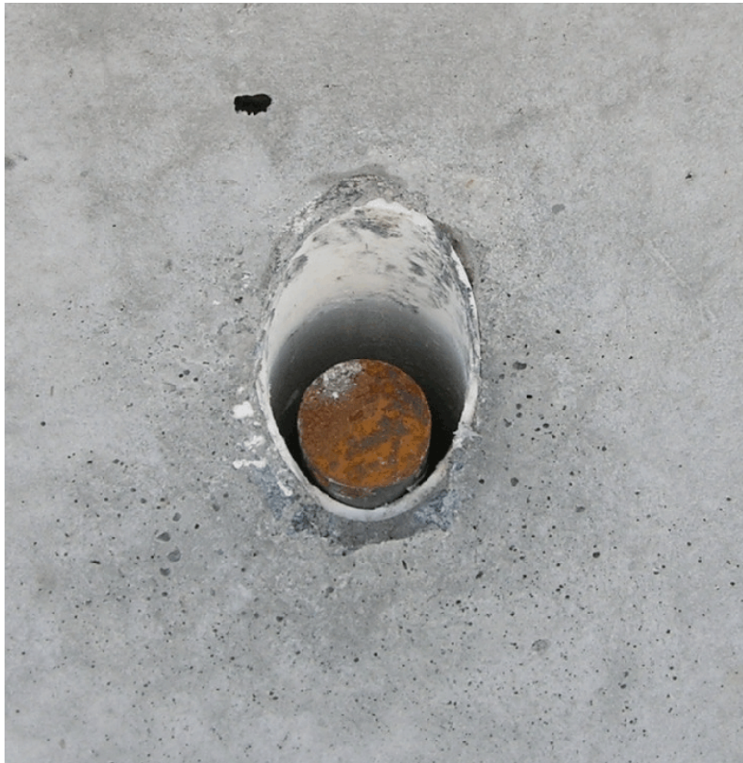
Figure 28. Anchored Barrier Ends, Test NYTCB-1
