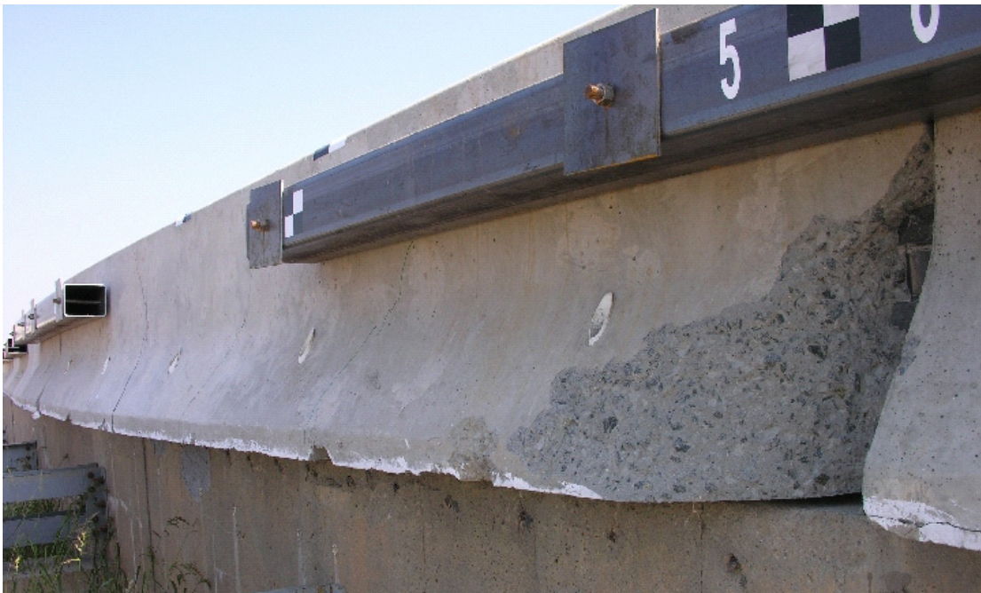
Figure 81. Box Beam Stiffened Temporary Barrier Damage, Test NYTCB-3
