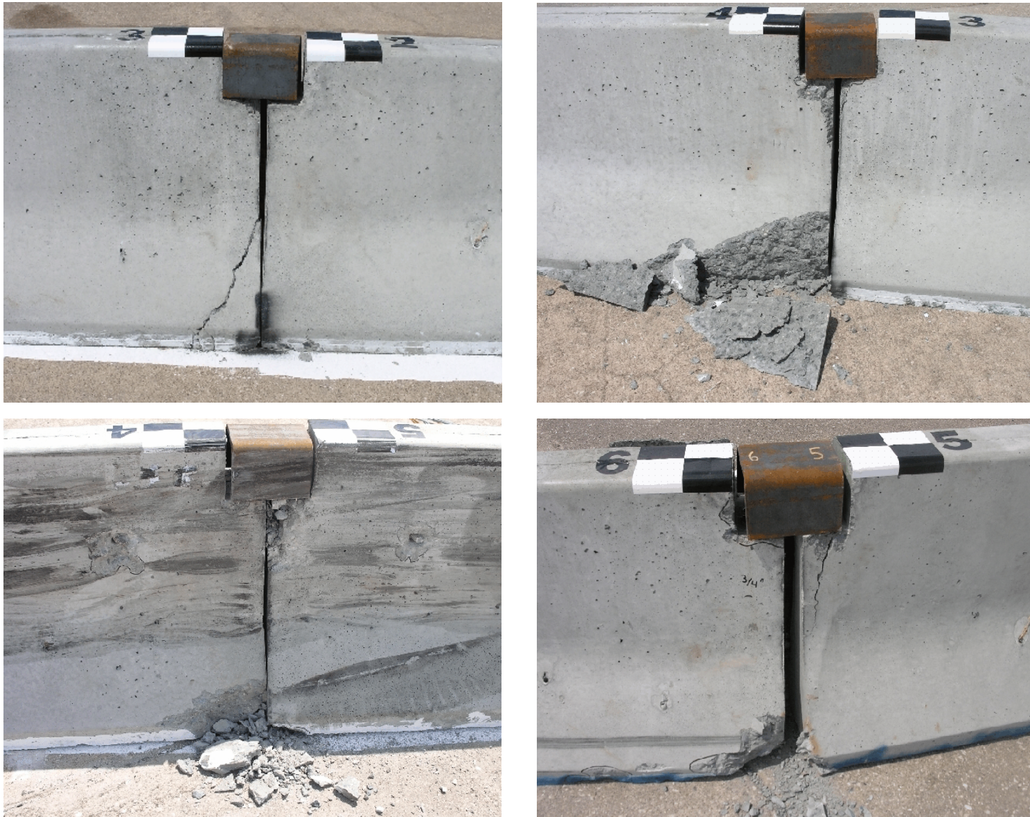
Figure 40. Joint Connection Damage - Joints 2-3, 3-4, 4-5, and 5-6, Test NYTCB-1
