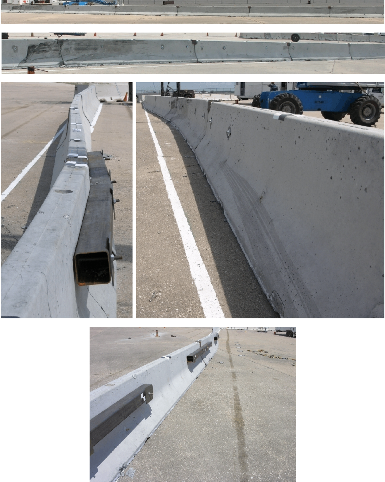
Figure 38. Temporary Barrier Damage, Test NYTCB-1
