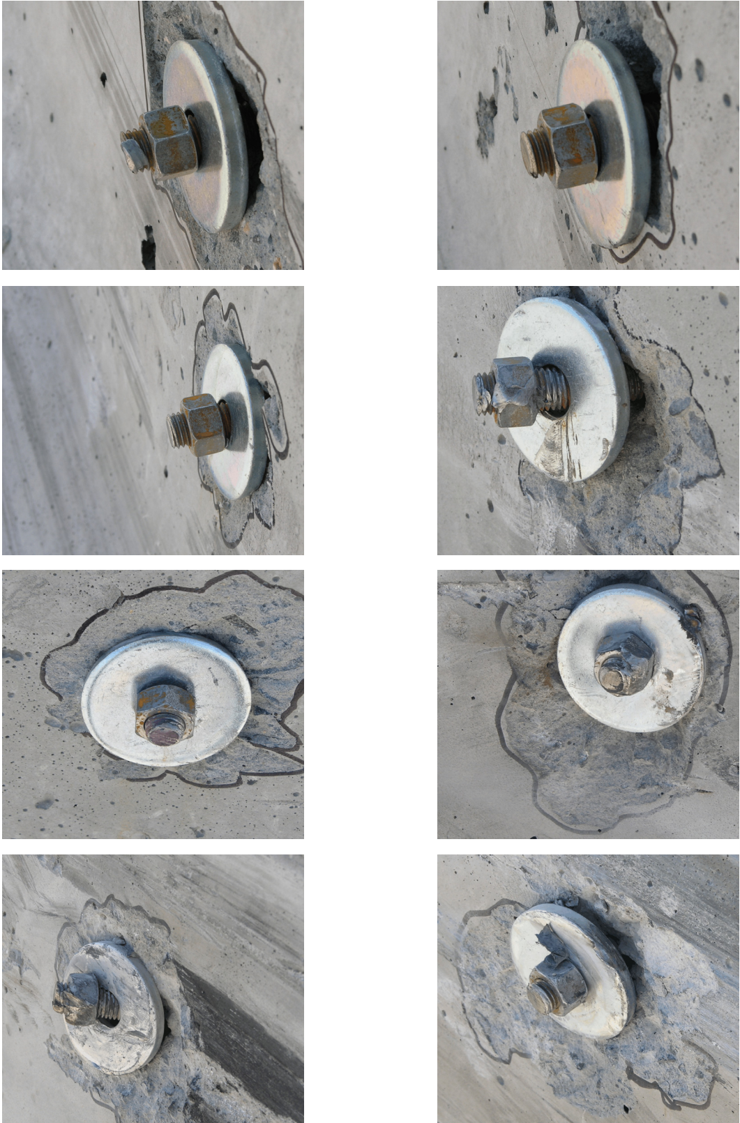
Figure 84. Connector Rod Damage, Test NYTCB-3
