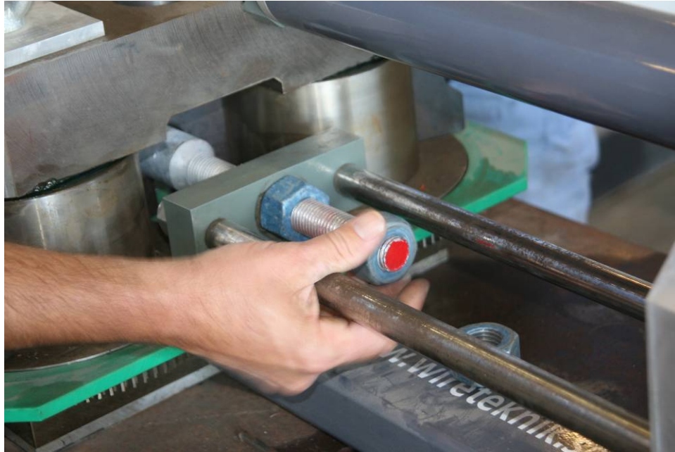
Figure 5. Image of Installation of Field Swage Termination in Swaging Machine.
