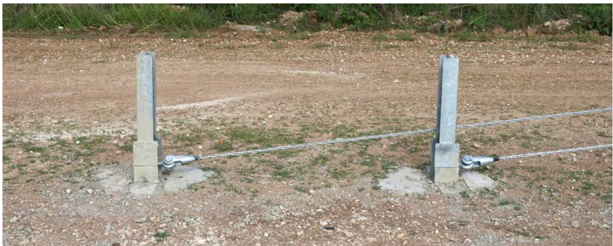
Figure 5.9. Retrofitted Low-tension wire rope barrier system prior to testing.
