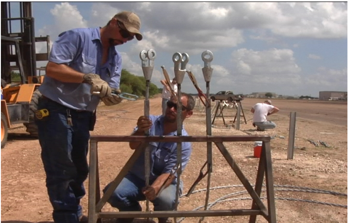
Figure 13. Suggested Method of Supporting Termination During Initial Curing Process.
