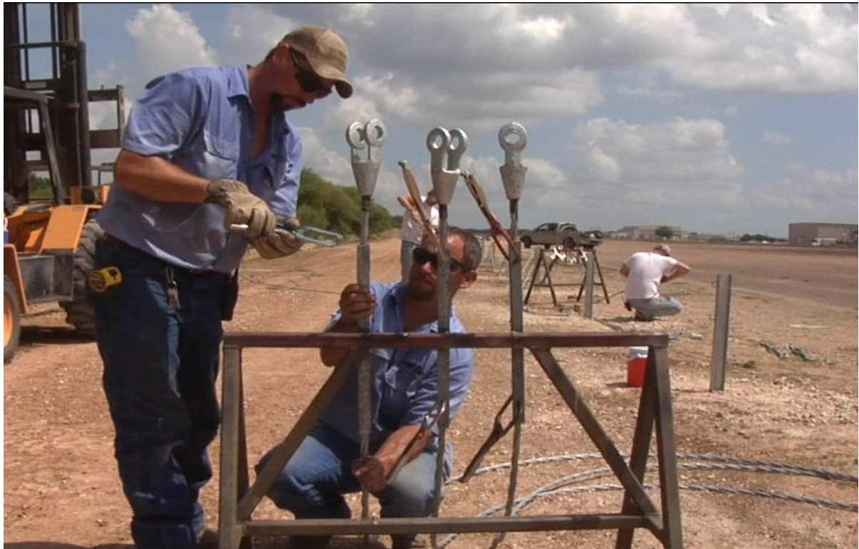
Figure 15. Suggested Method of Supporting Termination During Initial Curing Process.
