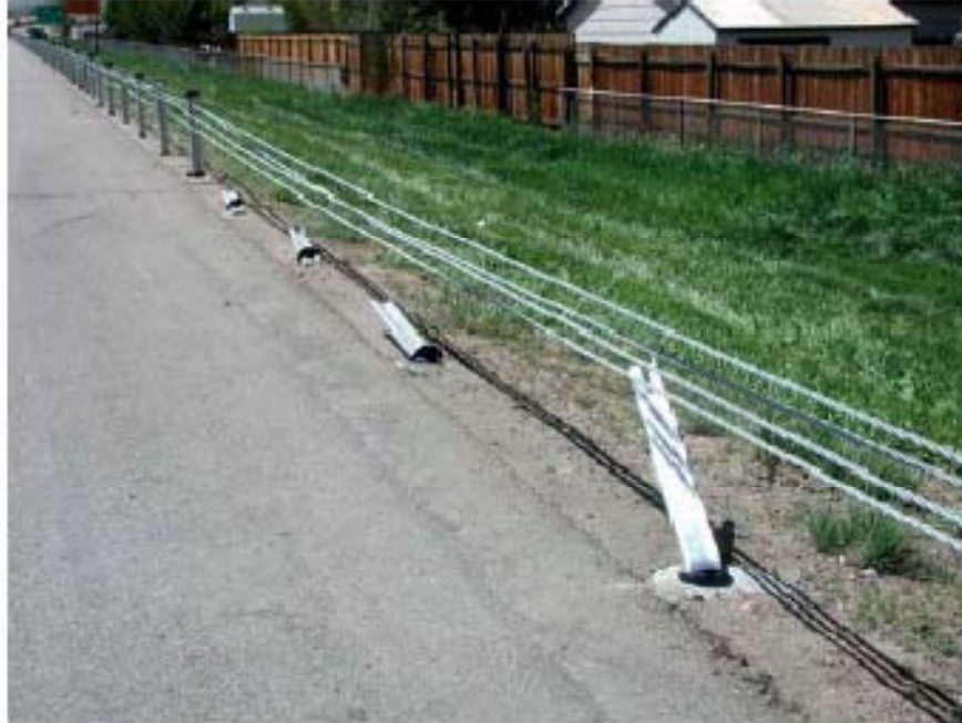
Figure 4.2. Image showing a high tension system after being impacted. (6)
