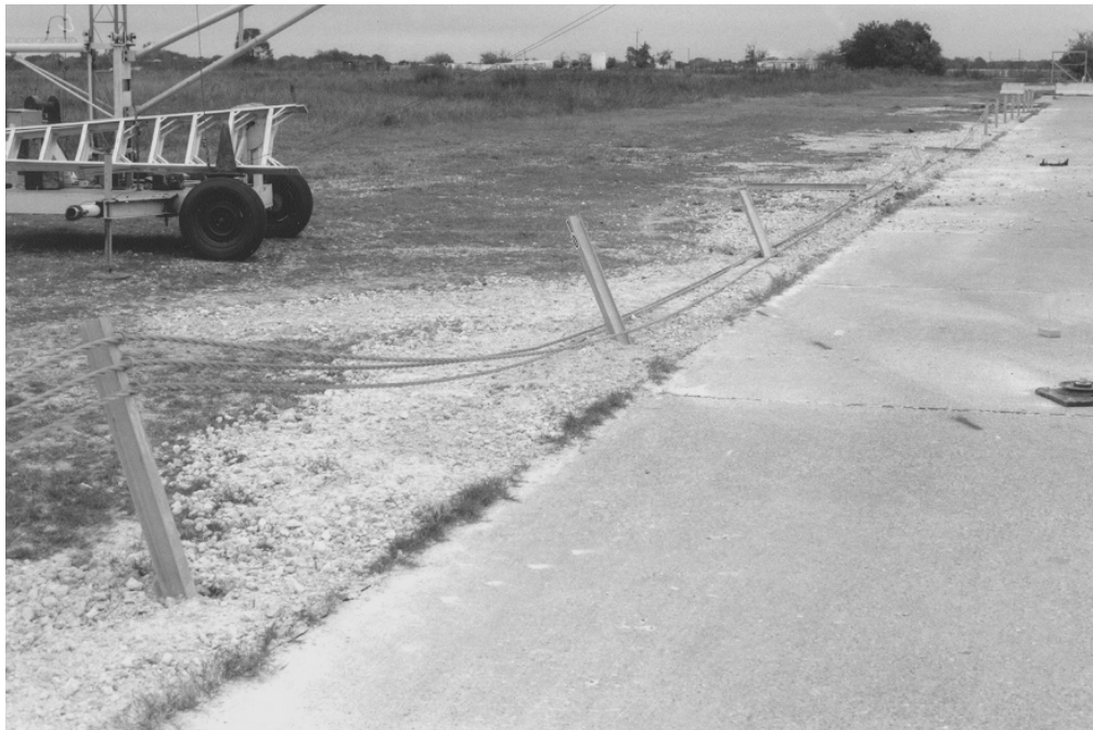
Figure 4.1. Image showing a low tension system after being impacted. (5)
