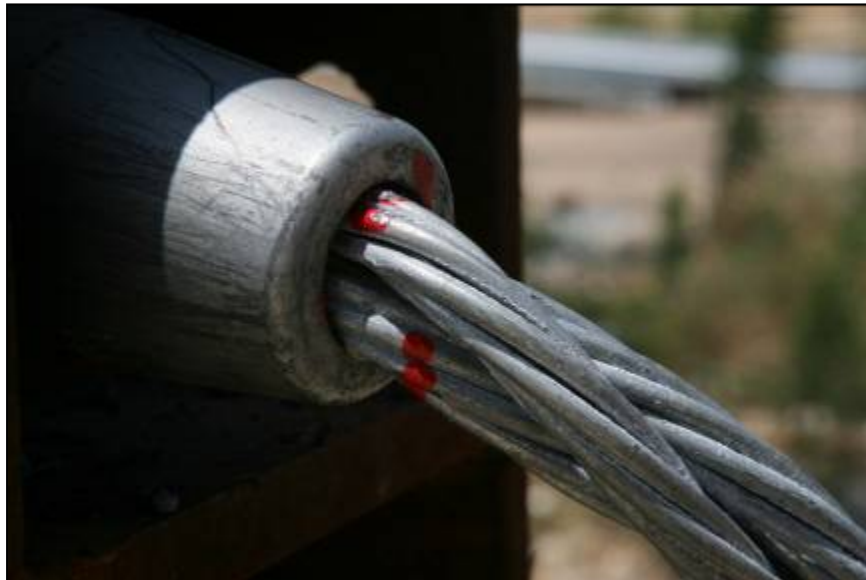
Figure 3.33. Nucor Steel Marion wire rope termination B after test NSM-P16.
