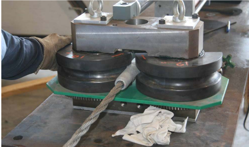
Figure 7. Image of a Proper Hand Placement during Wire Rope Swaging Process.
