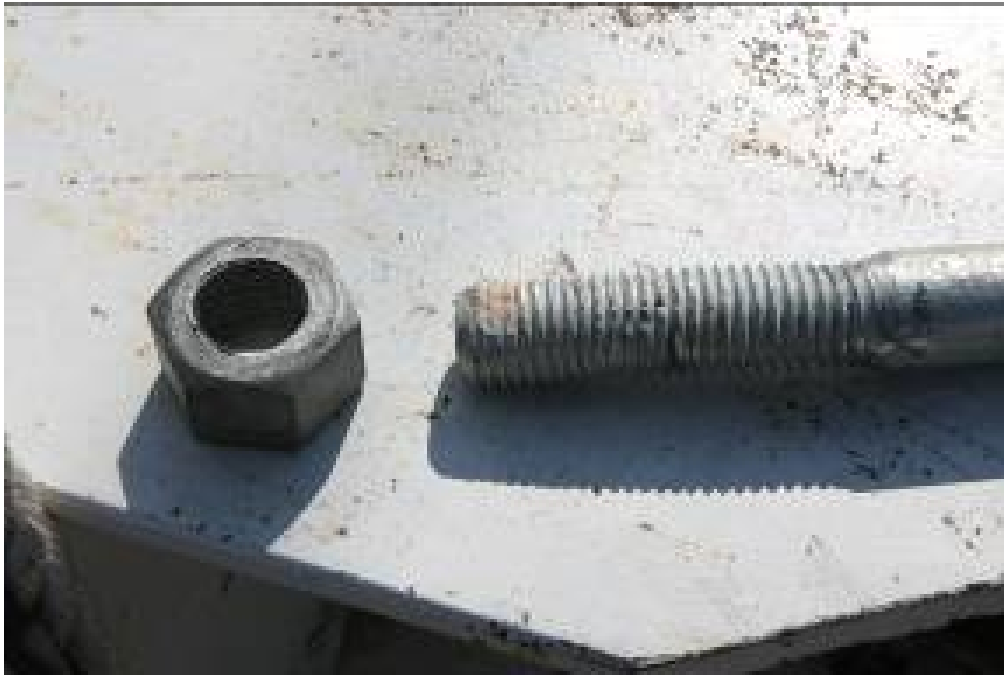
Figure 3.23. Epoxy Socket eyebolt and nut with stripped threads.
