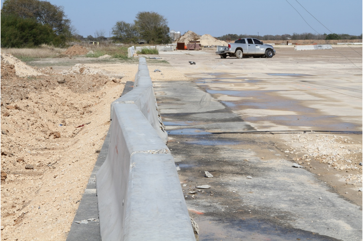
Figure 6.3. Vehicle and installation positions after test 405160-25-1.
