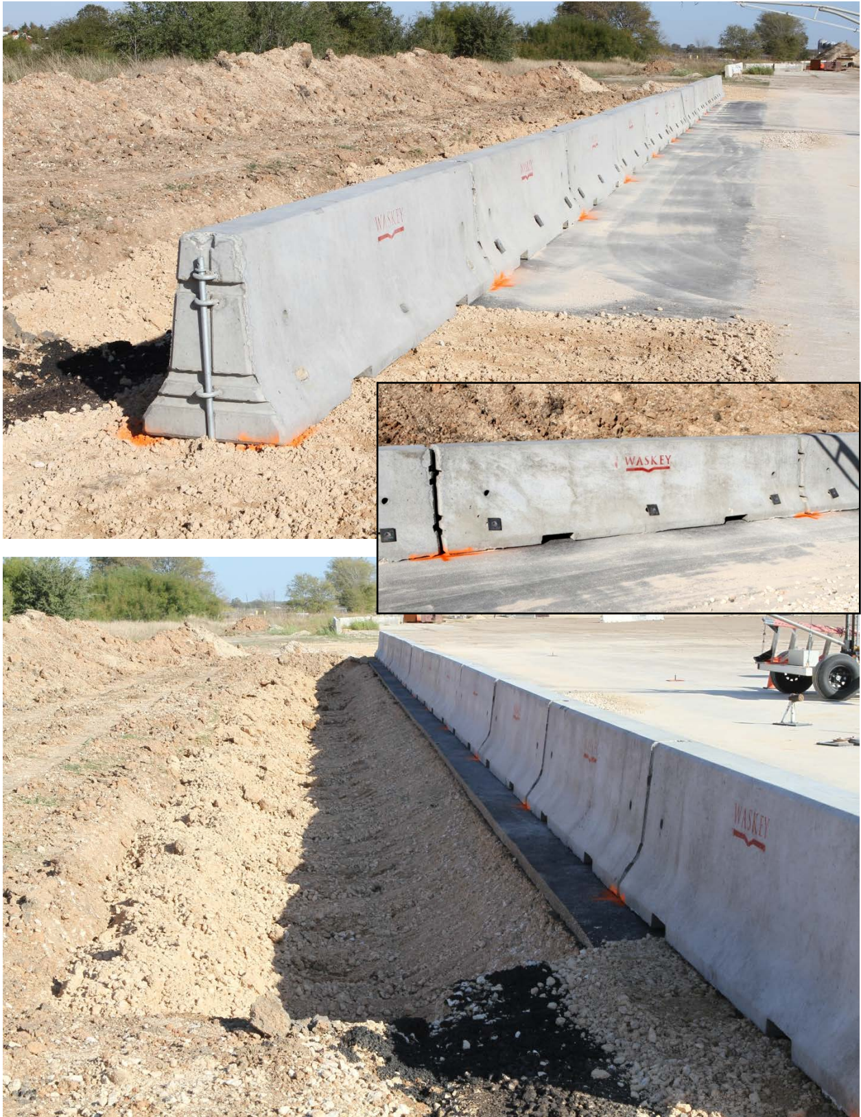
Figure 3.8. Temporary concrete barrier pinned on asphalt prior to testing.
