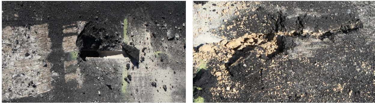
Figure 2.4. Tear in asphalt pad due to pin pullout. 4-inch pad (left), 2-inch pad (right).
