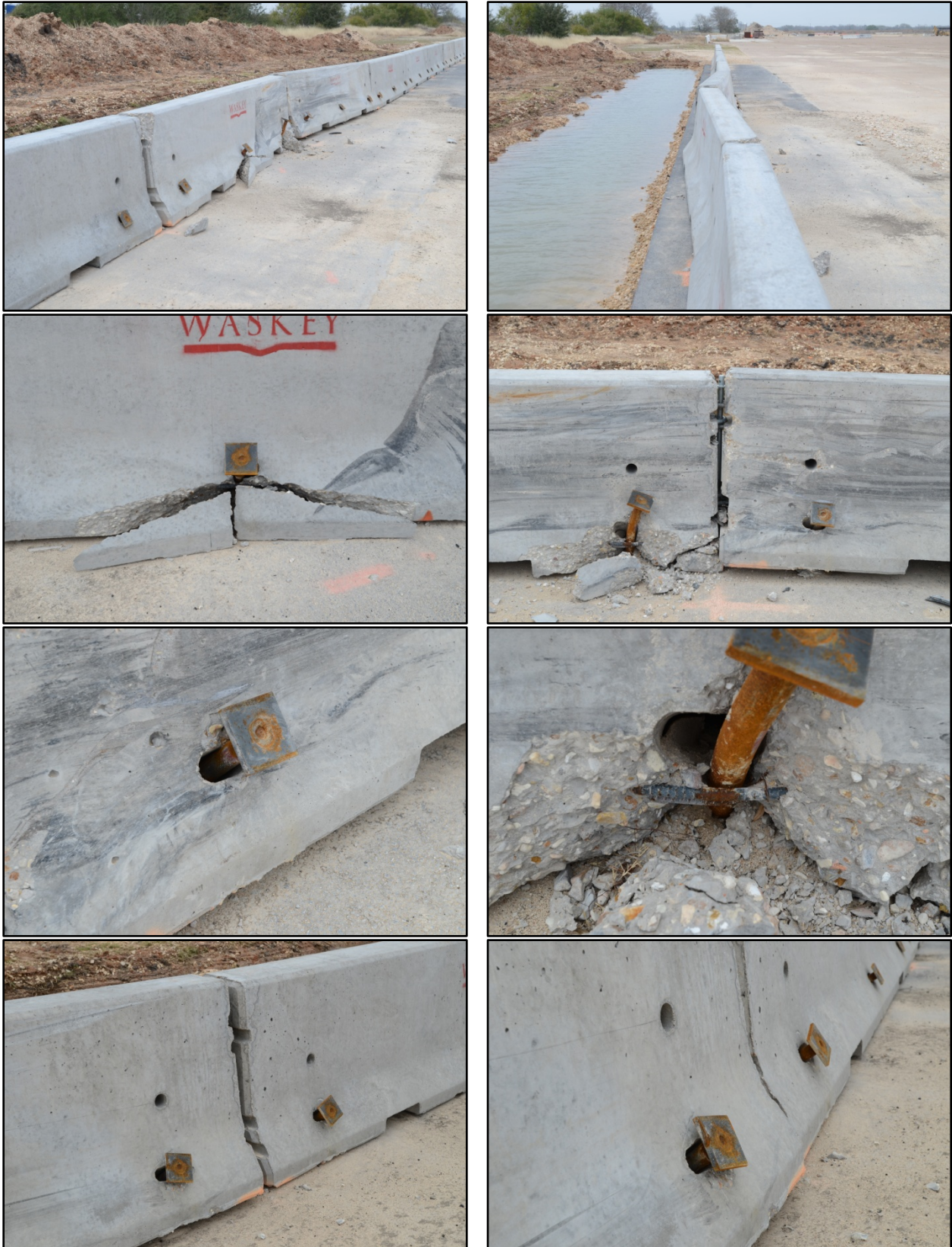
Figure 6.4. Installation after test 405160-25-1.
