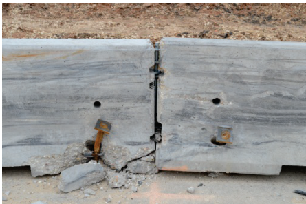
Pinned barrier after test
