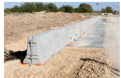
CMB pinned to asphalt
