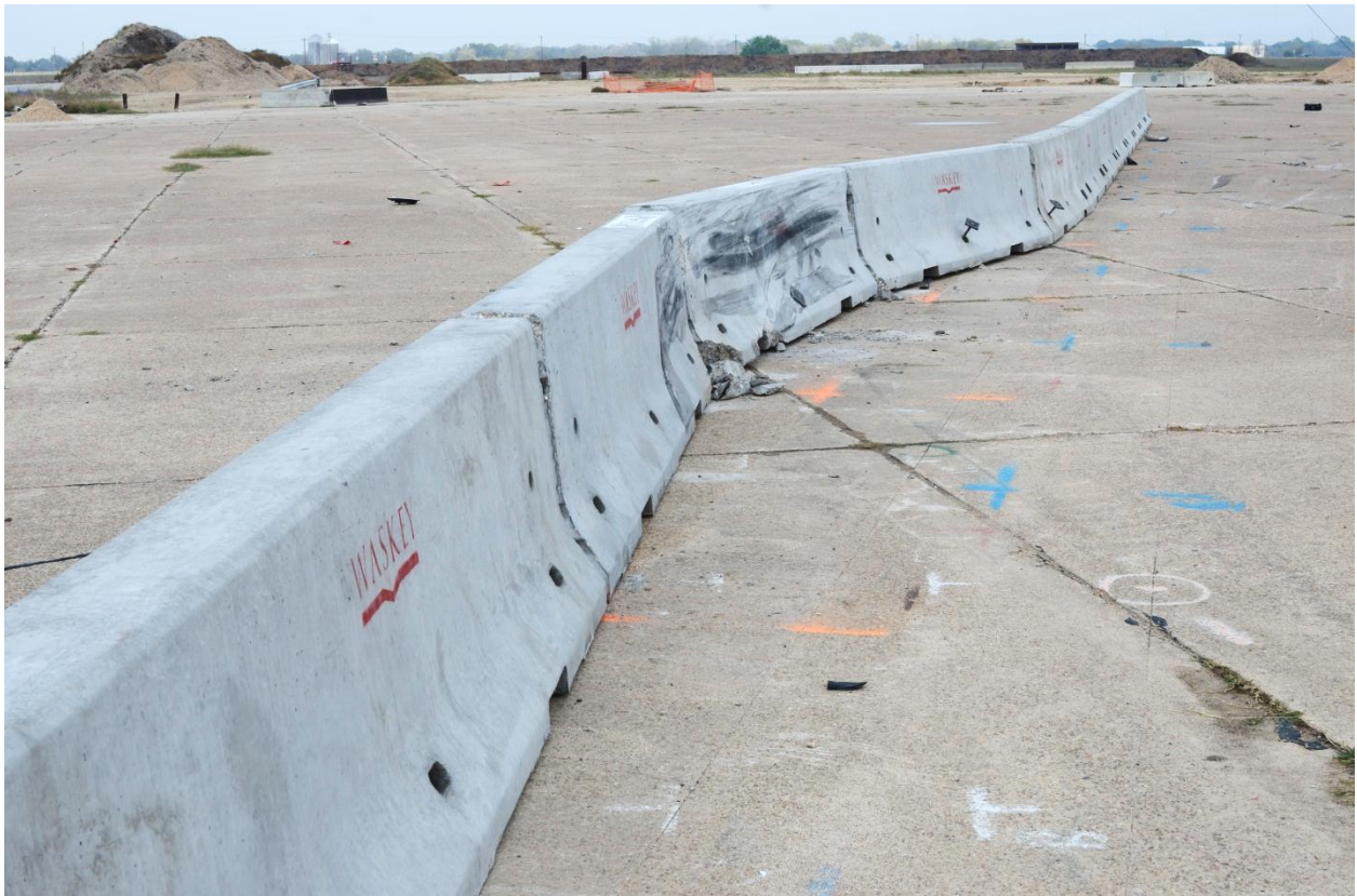
Figure A.6. Installation after test 405160-26-1.
