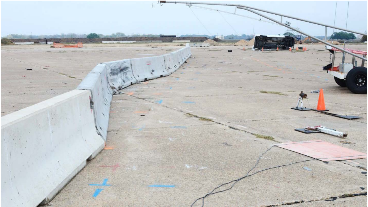
Figure A.5. Vehicle/installation positions after test 405160-26-1.
