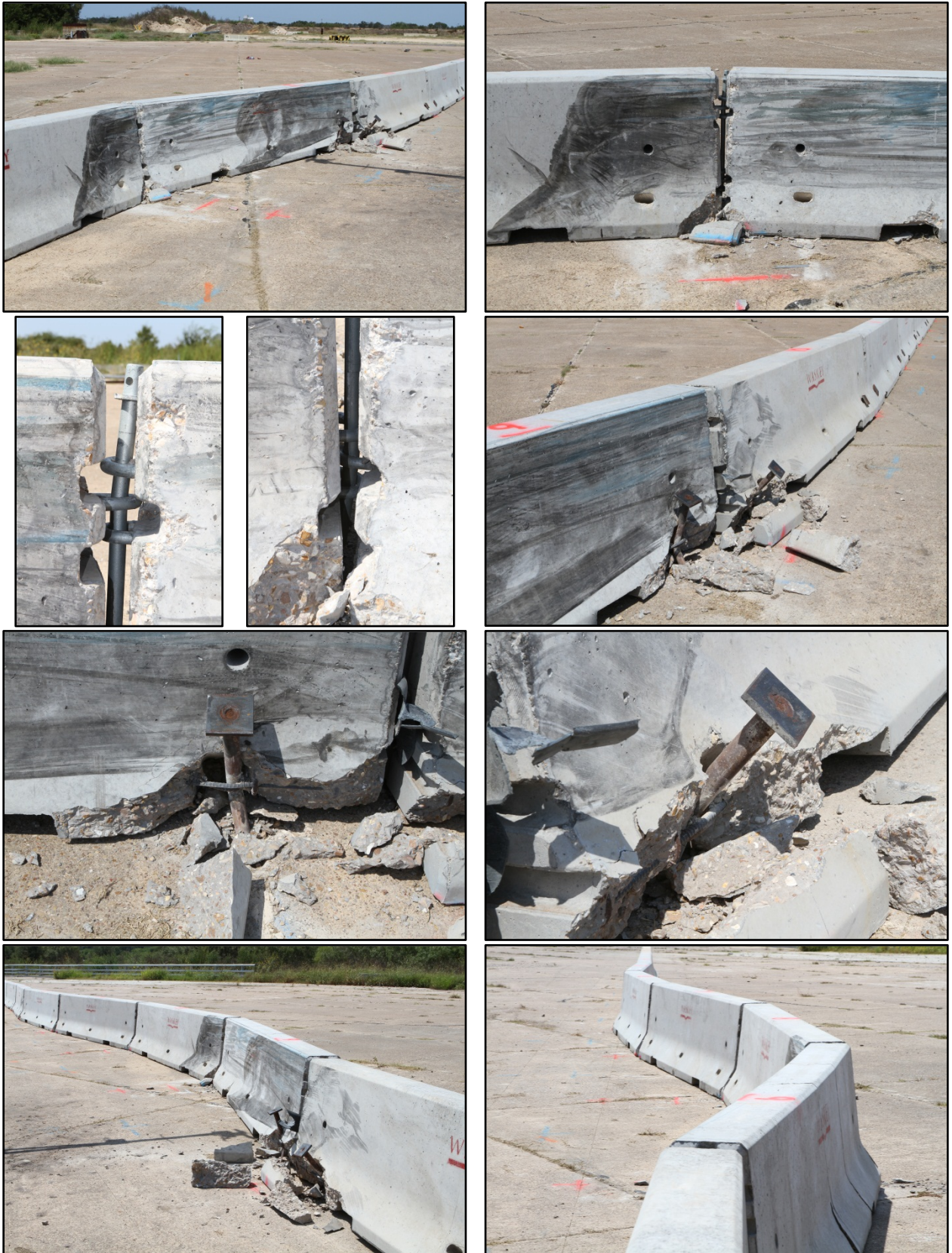
Figure 5.6. Installation after test 405160-26-2.
