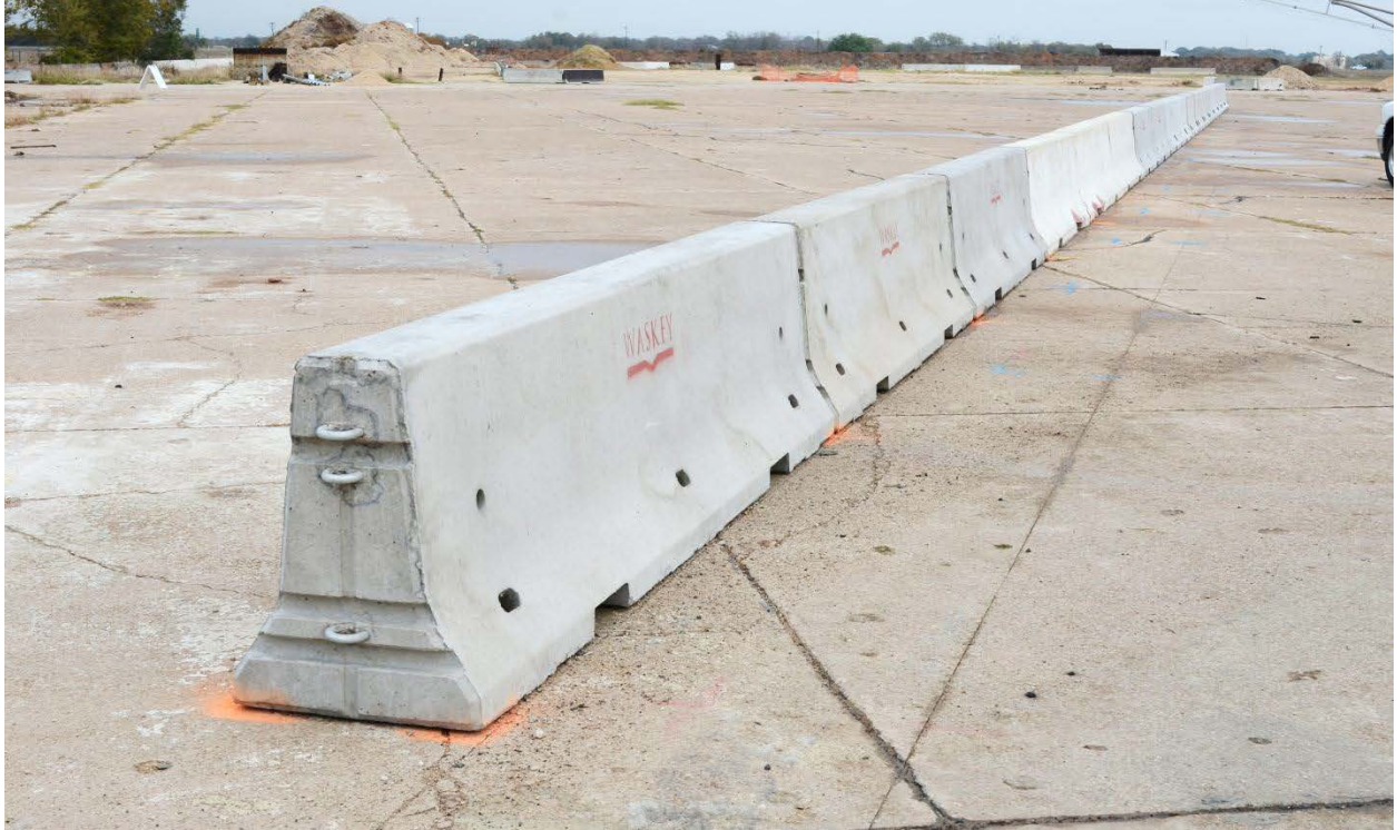
Figure A.2. Transition from free-standing F-shape barrier to pinned F shape barrier prior to test 405160-26-1.
