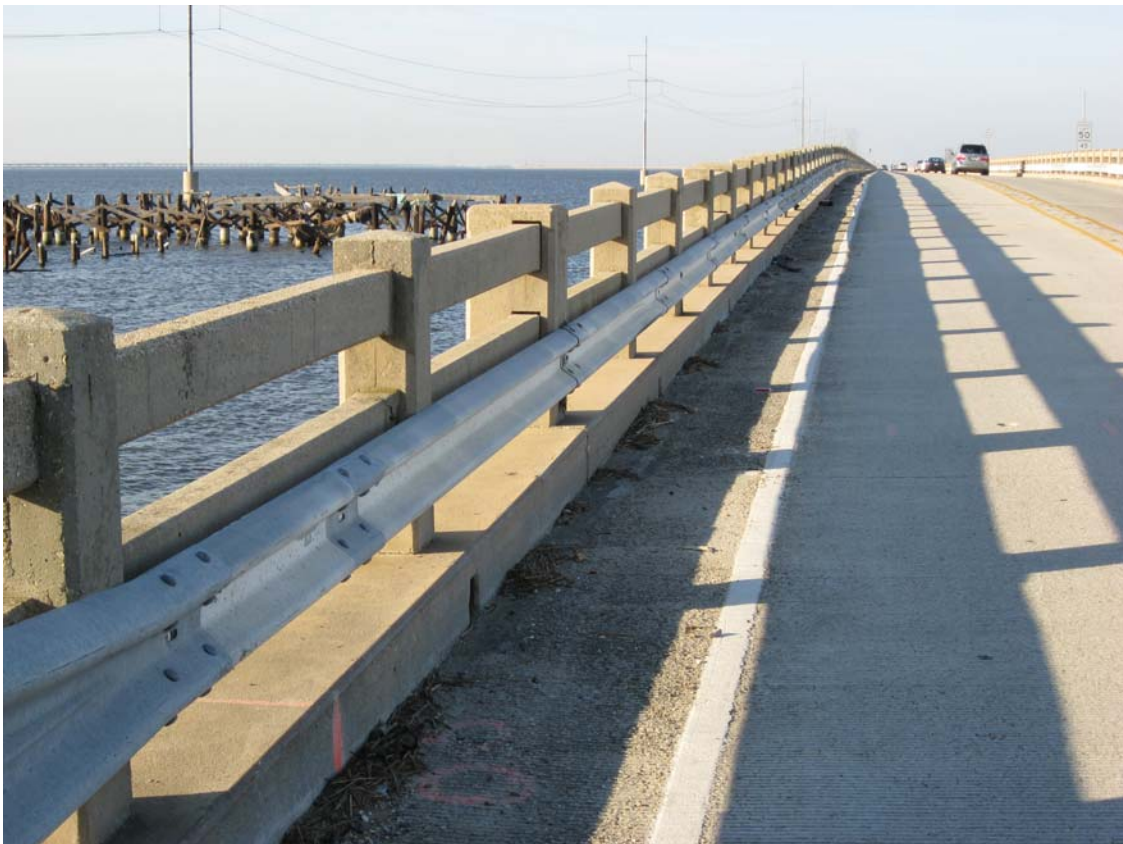
Figure 2 – Existing US 11 Lake Pontchartrain Bridge Rail Traffic Side View.
