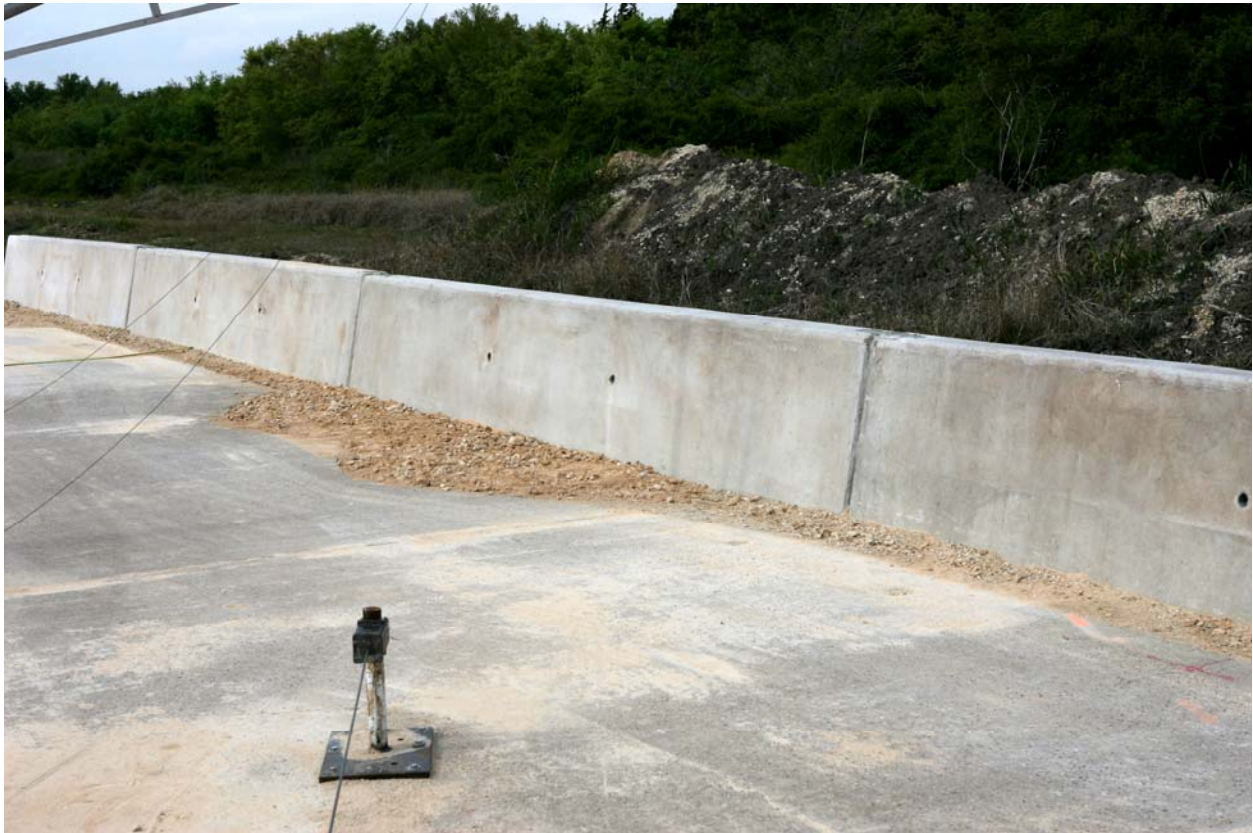
Figure 3.2. Single-slope barrier in front of 1.5:1 slope prior to testing.
