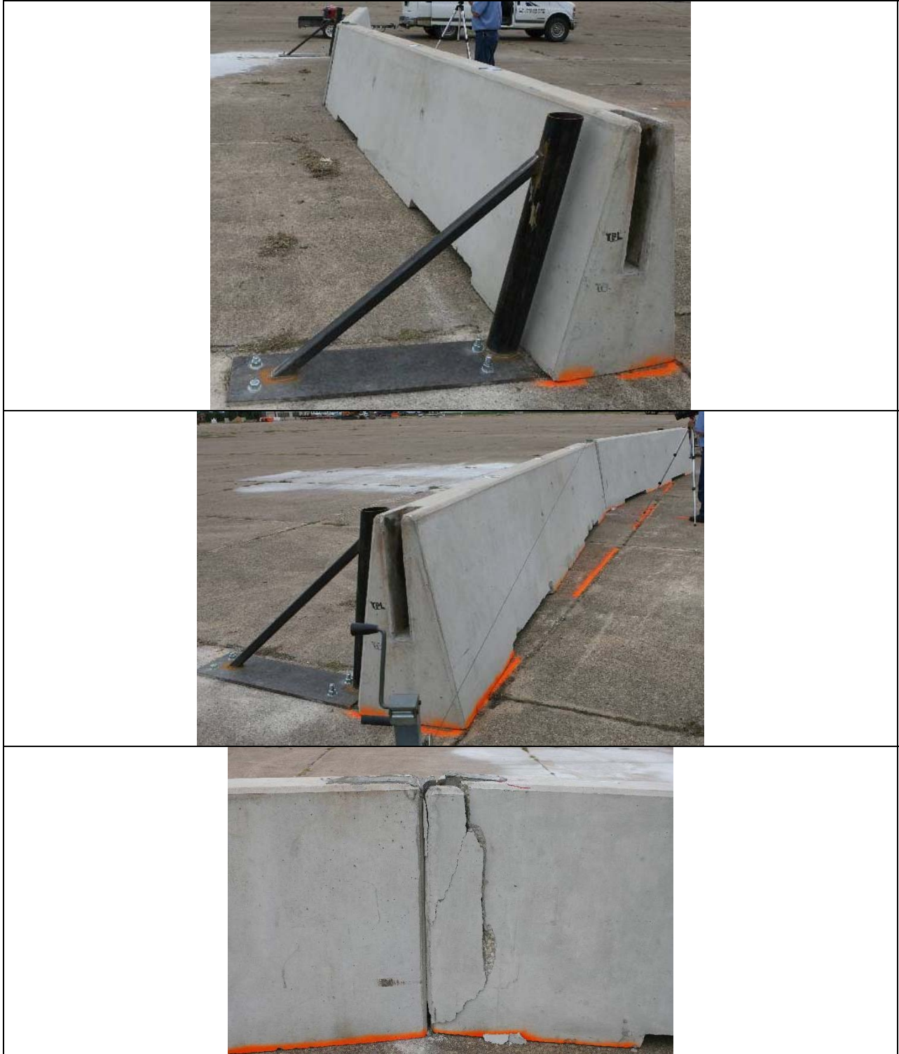
Figure 2.4. Barrier after impact from bogie vehicle.
