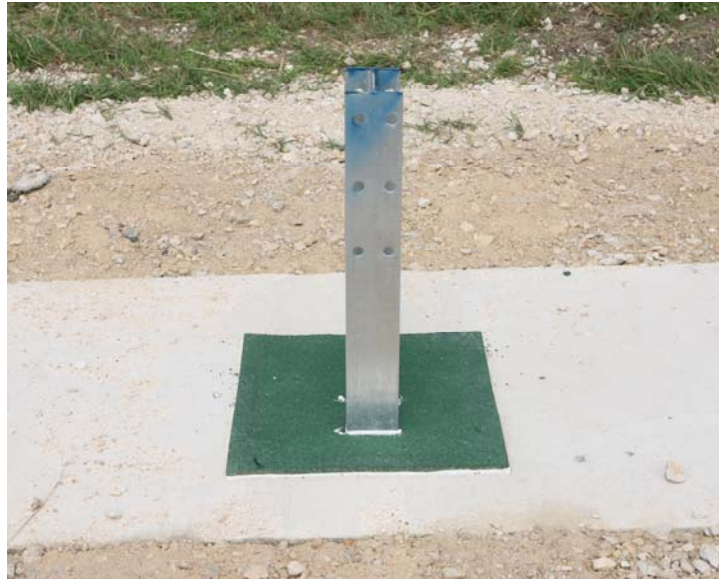
Figure 24: Post with TopHat™ recycled rubber mat prior to test B4.
