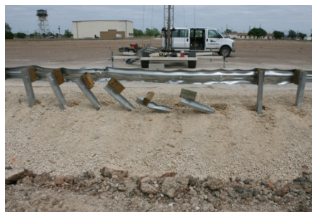
Barrier after Test
