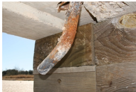
Damage to Drop Pin
