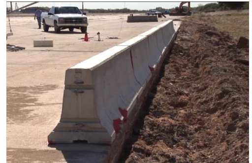
Test Installation of Pinned F-Shape Temporary Barrier
