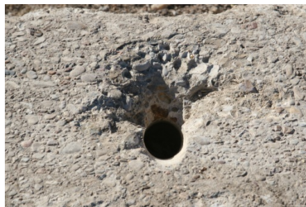
Damage to Drilled Hole
