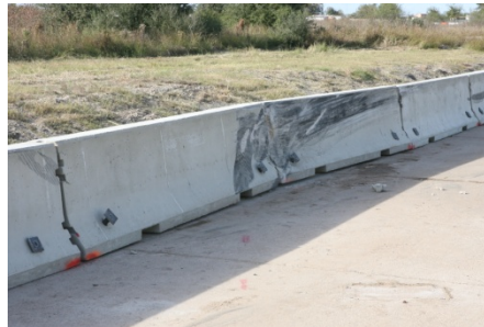
Barrier after Test
