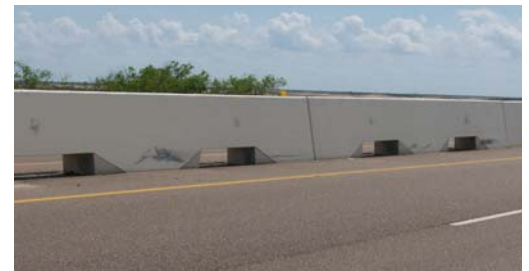
TXDOT Single Slope Concrete Barrier (Wildlife Crossing) SSCB
