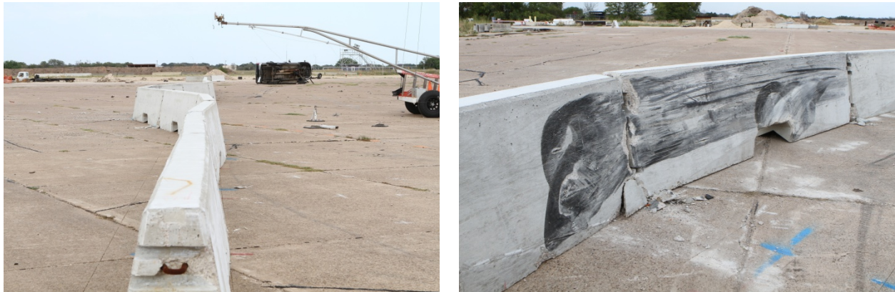
Figure 2. Damage to WSDOT pin and loop barrier with drainage slots after test 405160-30-1.
