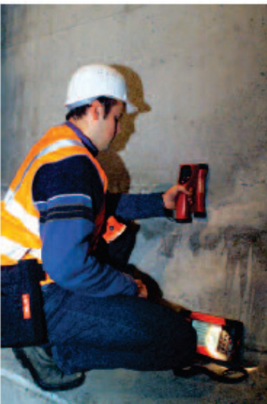
Quickscan for localizing reinforcement bars
