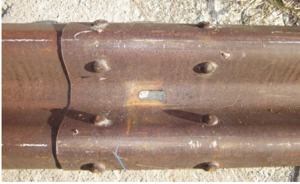
California W-beam rail splice
