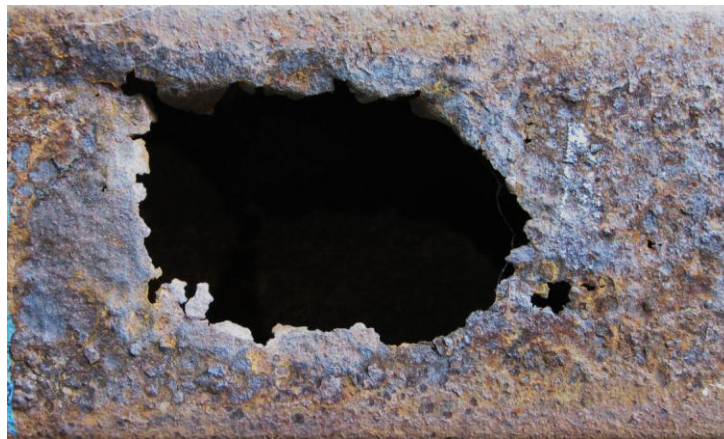
Figure 3.3 Advanced rail corrosion with pitting.
