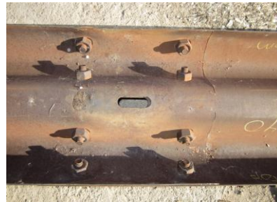
Mark spot 2: Field side splice bolt (post not shown)
