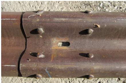
Mark spot 1: Traffic side splice bolt
