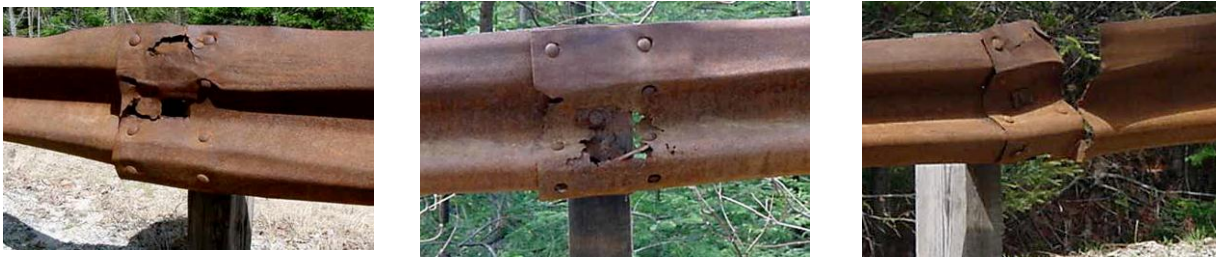
Figure 4.1: Examples of failed guardrails that can be visually identified.
