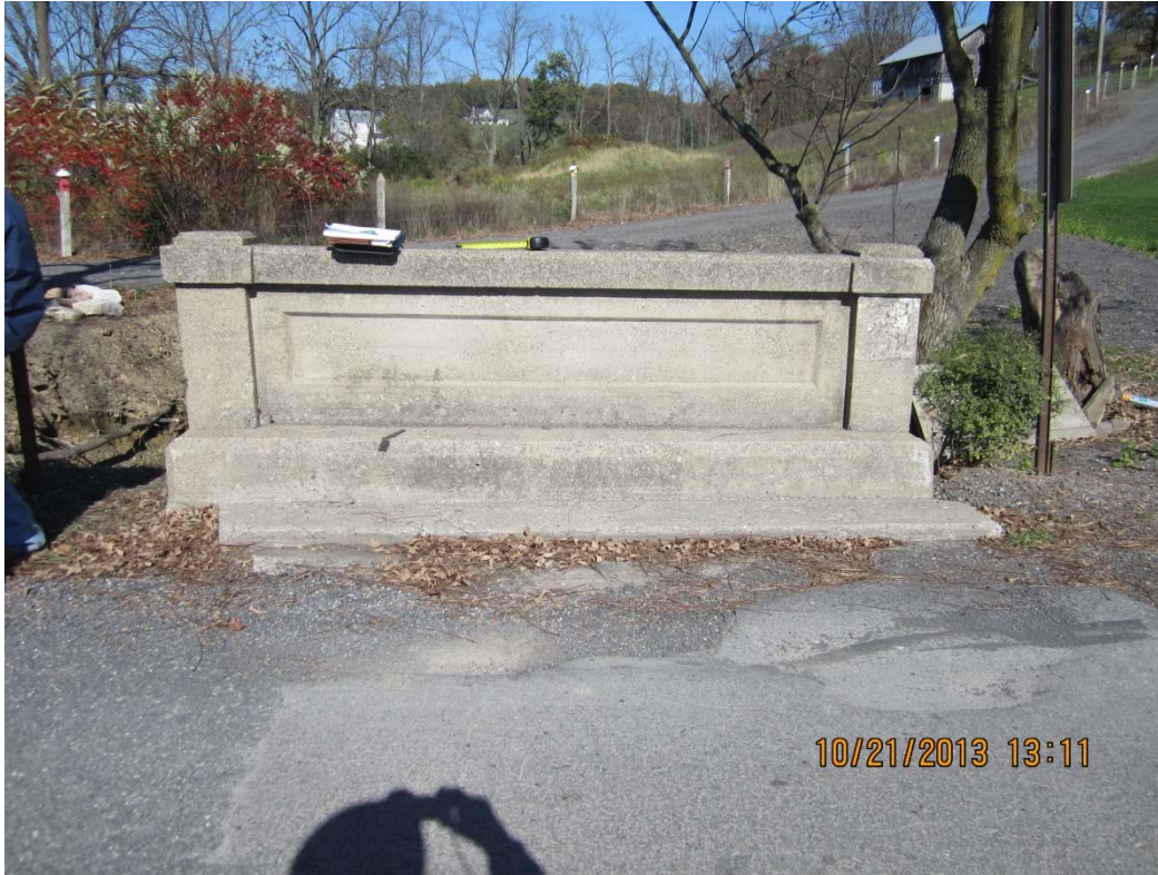
Figure 15 – Photo of Typical Concrete Parapet Without Openings
