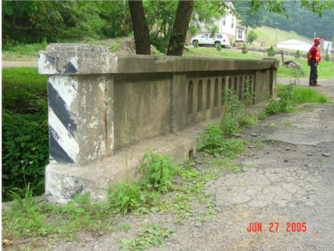
Figure 4 – Typical Photo of Concrete Post and Beam Railing with Concrete Pickets
