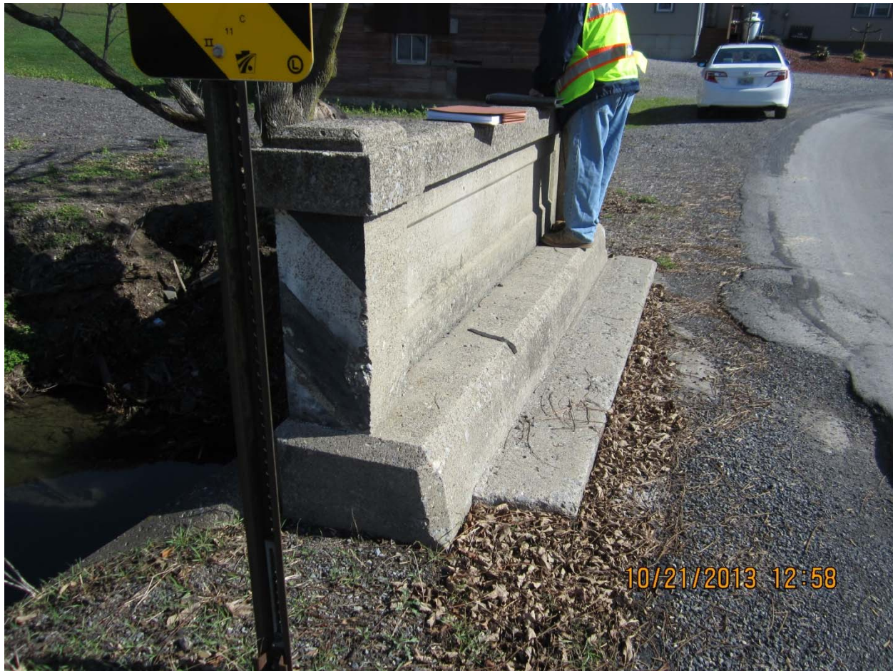
Figure 16 – Photo of Typical Concrete Parapet Without Openings
