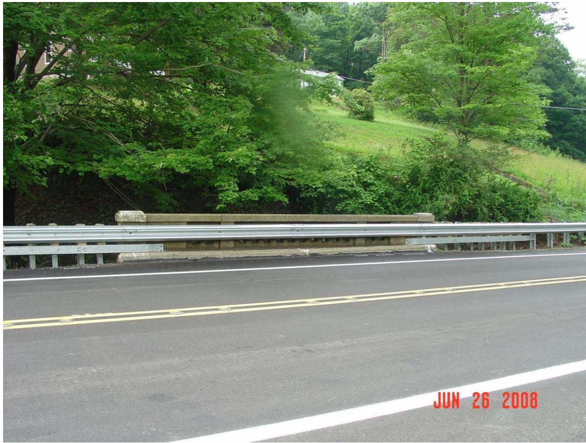
Figure 10 – Front View of Retrofit Option Using W-Beam Guardrail
