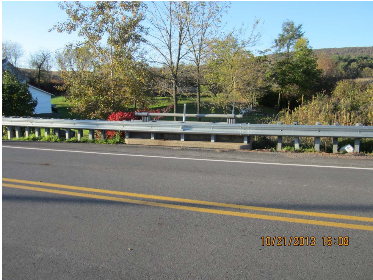
Figure 22 – Photo of Combination Concrete Rail with Aluminum Post and Rail
