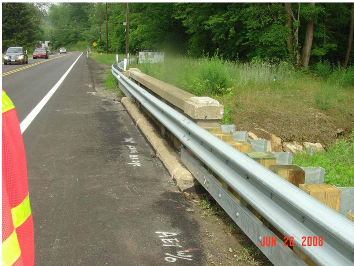
Figure 9 – Retrofit Option Using W-Beam Guardrail
