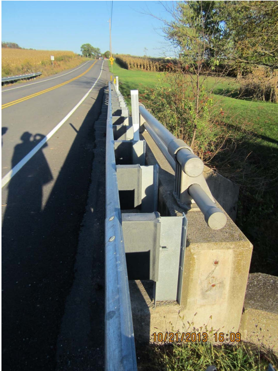
Figure 23 – Photo of Combination Concrete Rail with Aluminum Post and Rail
