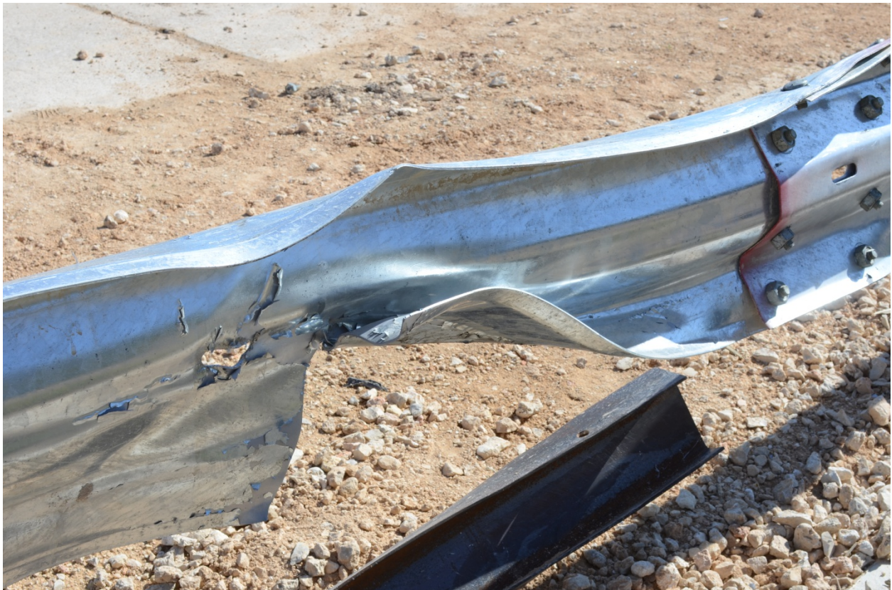
Figure 5.4. Installation after test 405160-23-2.
