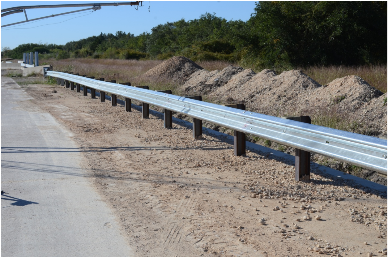
Figure 2.2. W-Beam Guardrail on Low-Fill Box Culvert prior to testing.
