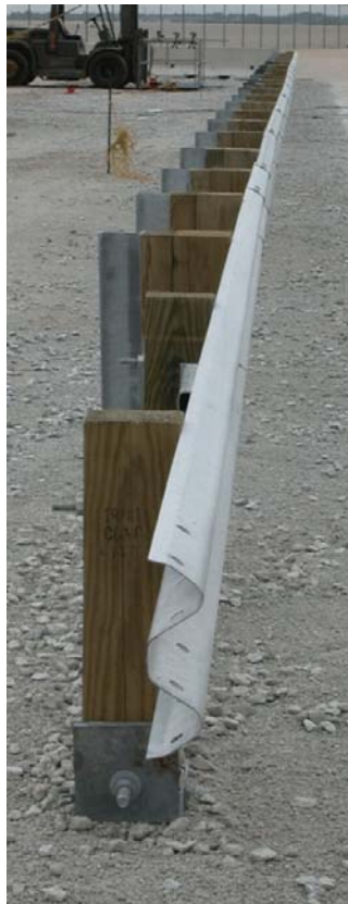
Figure 11. Midwest Guardrail System
