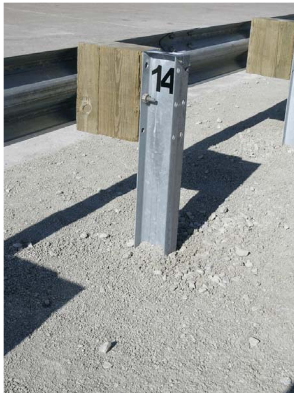
Figure 12. Midwest Guardrail System - Maximum Height Tolerance
