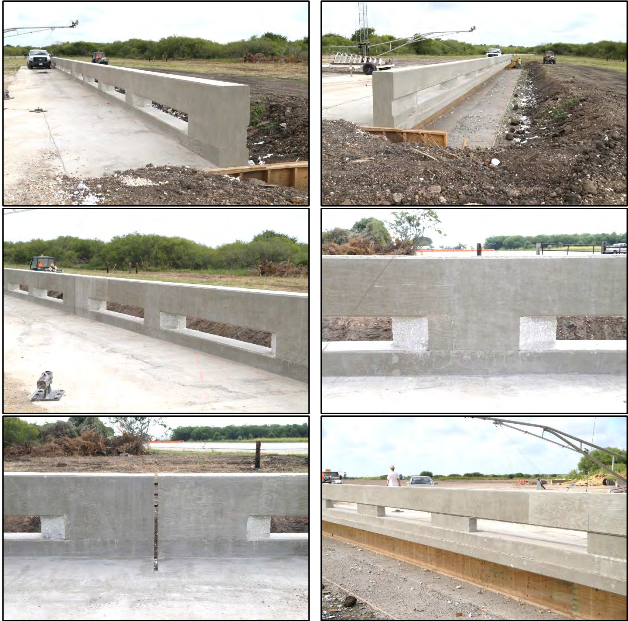
Figure 2.2. TxDOT T224 Bridge Rail prior to Testing.
