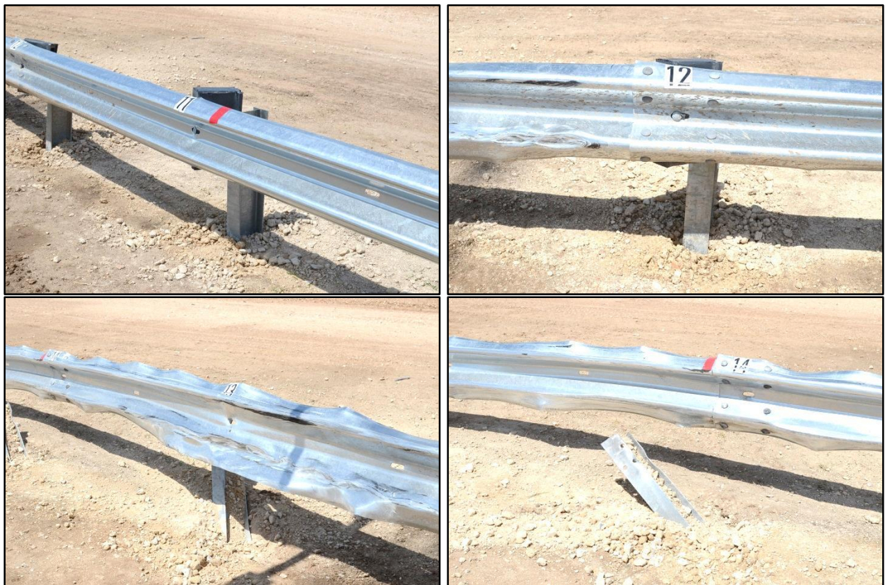
Figure 5.5. Posts 11 through 14 after Test No. 608421-1.
