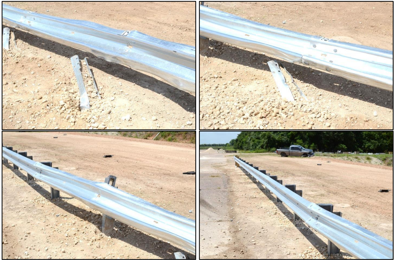
Figure 5.6. Posts 15 through 18 after Test No. 608421-1.
