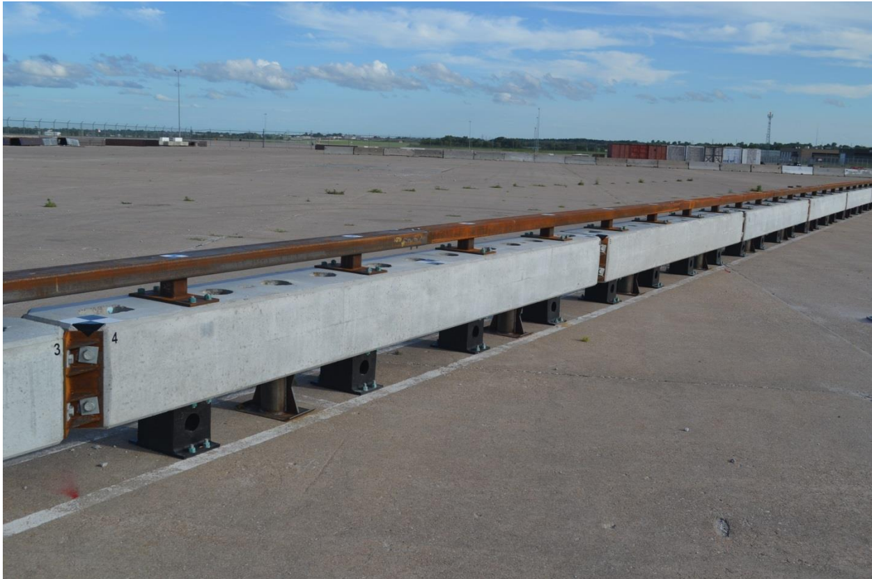
Figure 1. View of Initial Concept with Rubber Posts and Metal Skids [3]
