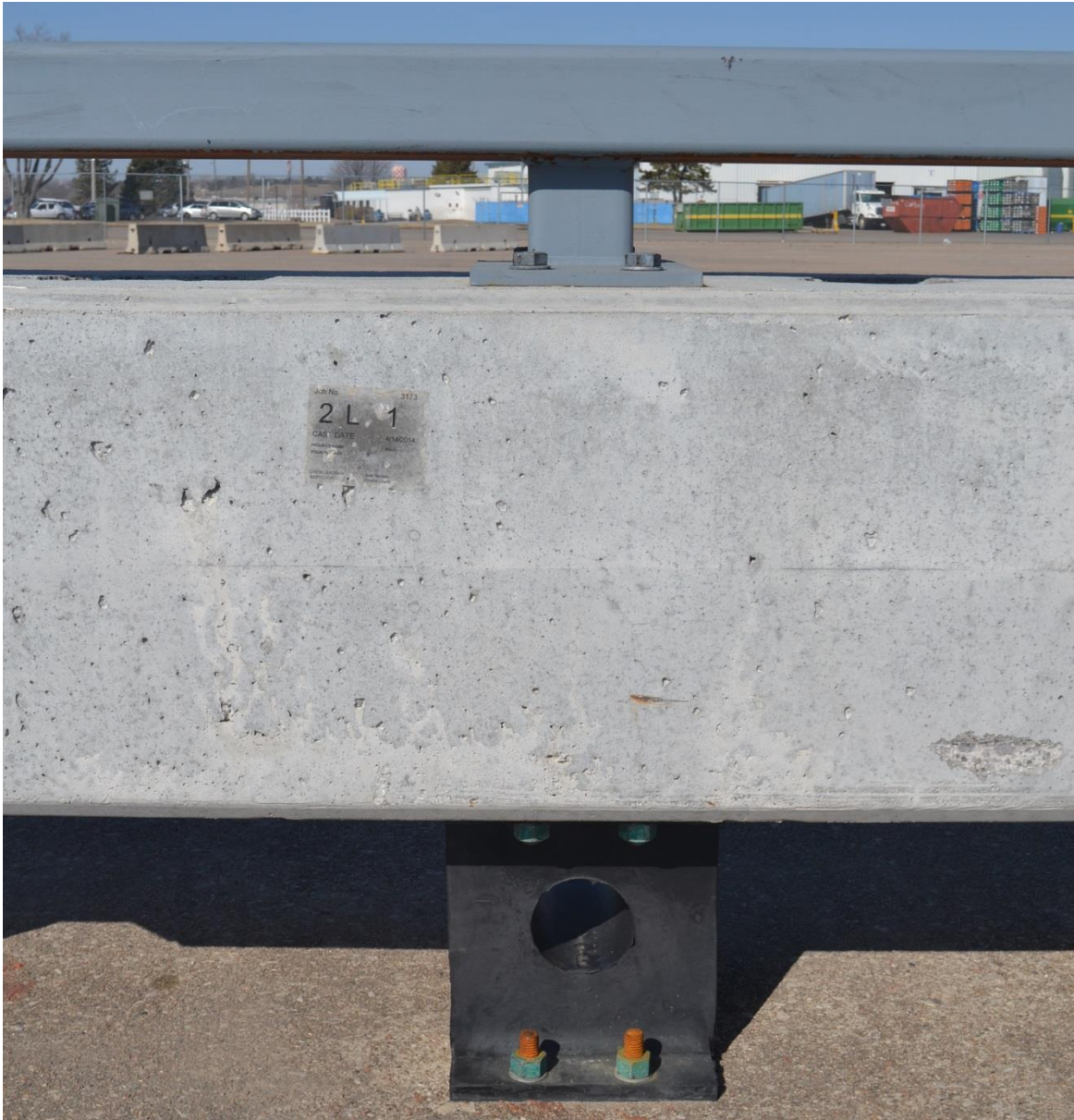
Figure 102. Upper Rail Assembly thru Bolt Connection, Test No. SFH-3
