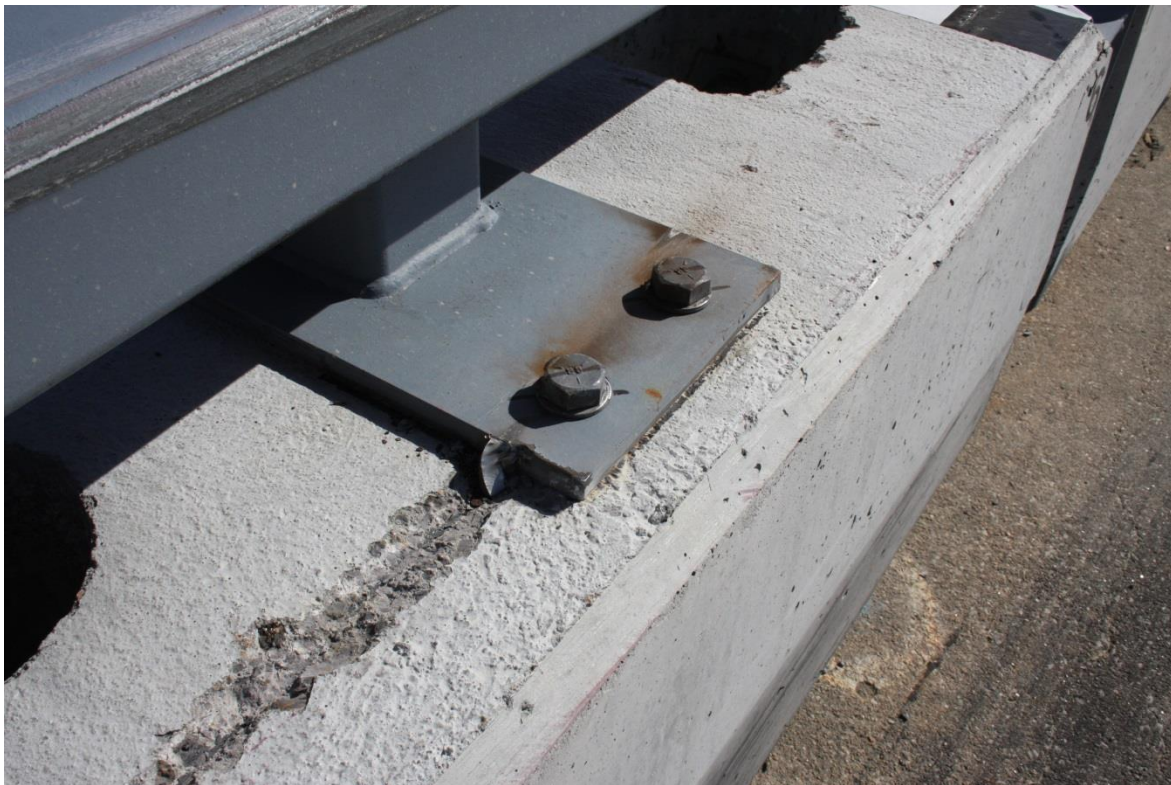
Figure 115. System Damage, First Upper Tube Assembly Connection Upstream from Joint between Barrier Nos. 6 and 7, Test No. SFH-3
