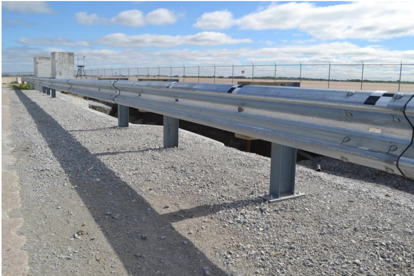
Figure 34. Test Installation, Test No. MGSLS-1
