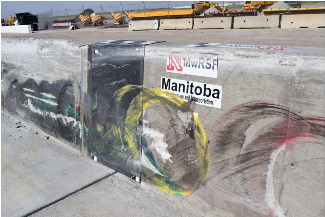
Figure 40. System Damage, Test No. MAN-1
