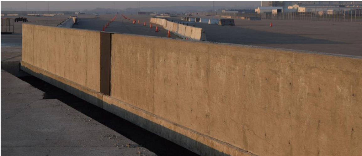
Figure 26. Test Installation Photographs, Test No. MAN-1
