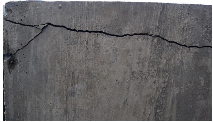
Bottom of deck, downstream of joint
