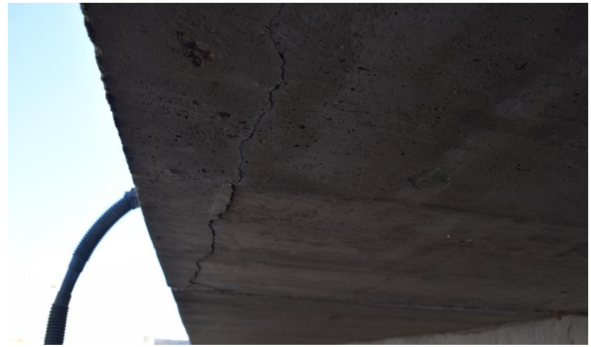
Bottom of deck, downstream of joint
