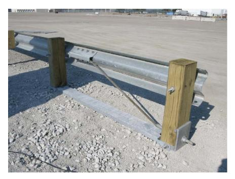
Figure 21. Approach Guardrail Transition to Concrete Barrier System
