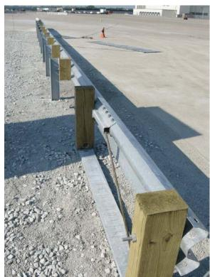
Figure 20. Approach Guardrail Transition to Concrete Barrier System
