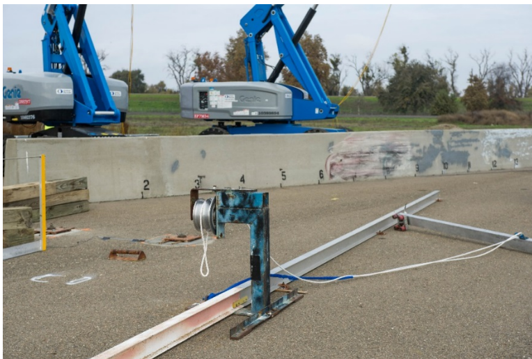
Figure 5-7 Type 60 Barrier Post Test Upstream of Impact
