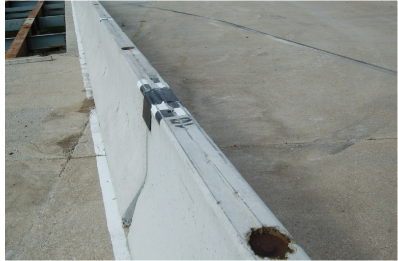
Joint between Barrier Nos. 9 and 10
