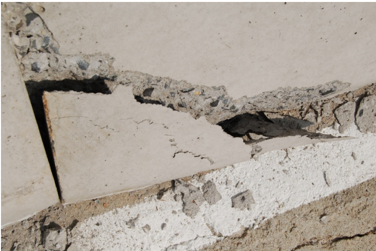
Figure 28. Barrier No. 4 Damage, Test No. NYTCB-5
