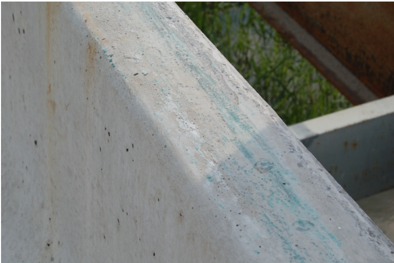
Figure 31. Barrier No. 8 Damage, Test No. NYTCB-5
