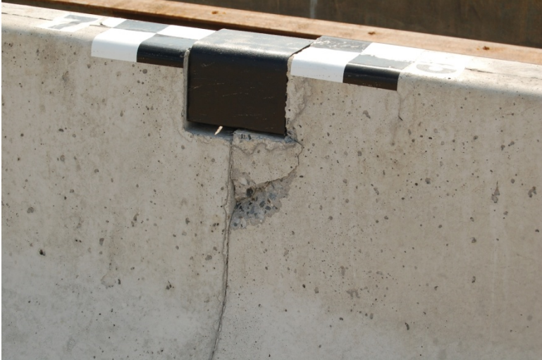
Joint between Barrier Nos. 6 and 7
