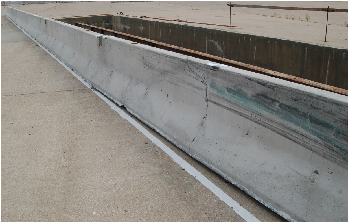
Figure 26. System Damage, Test No. NYTCB-5
