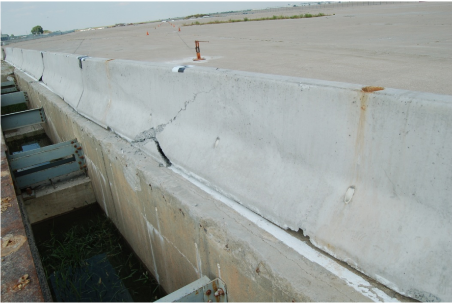
Figure 25. System Damage, Test No. NYTCB-5
