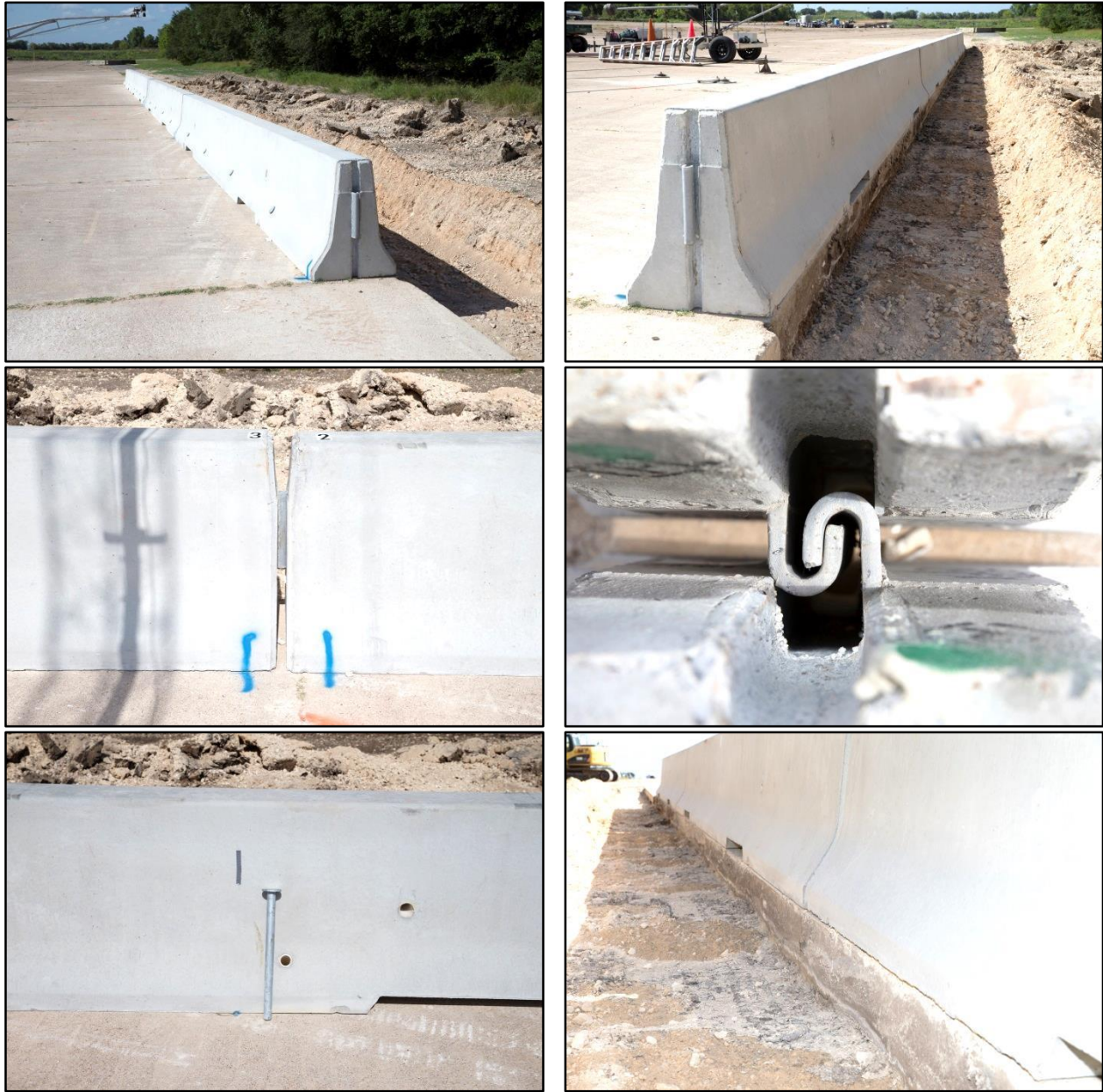
Figure 4.2. TxDOT 32-inch CSB(7)-10 Pinned to Concrete Pavement prior to Testing.
