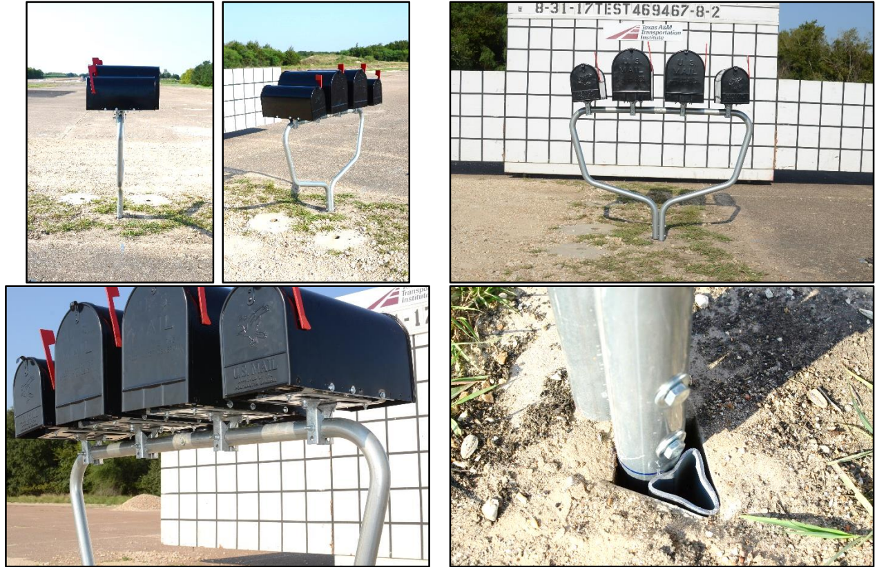
Figure 7.19. TxDOT Multiple Mailbox System on 56-inch Hanger-Type Thin-Walled Galvanized Tube with Type 1 Foundation prior to Testing.
