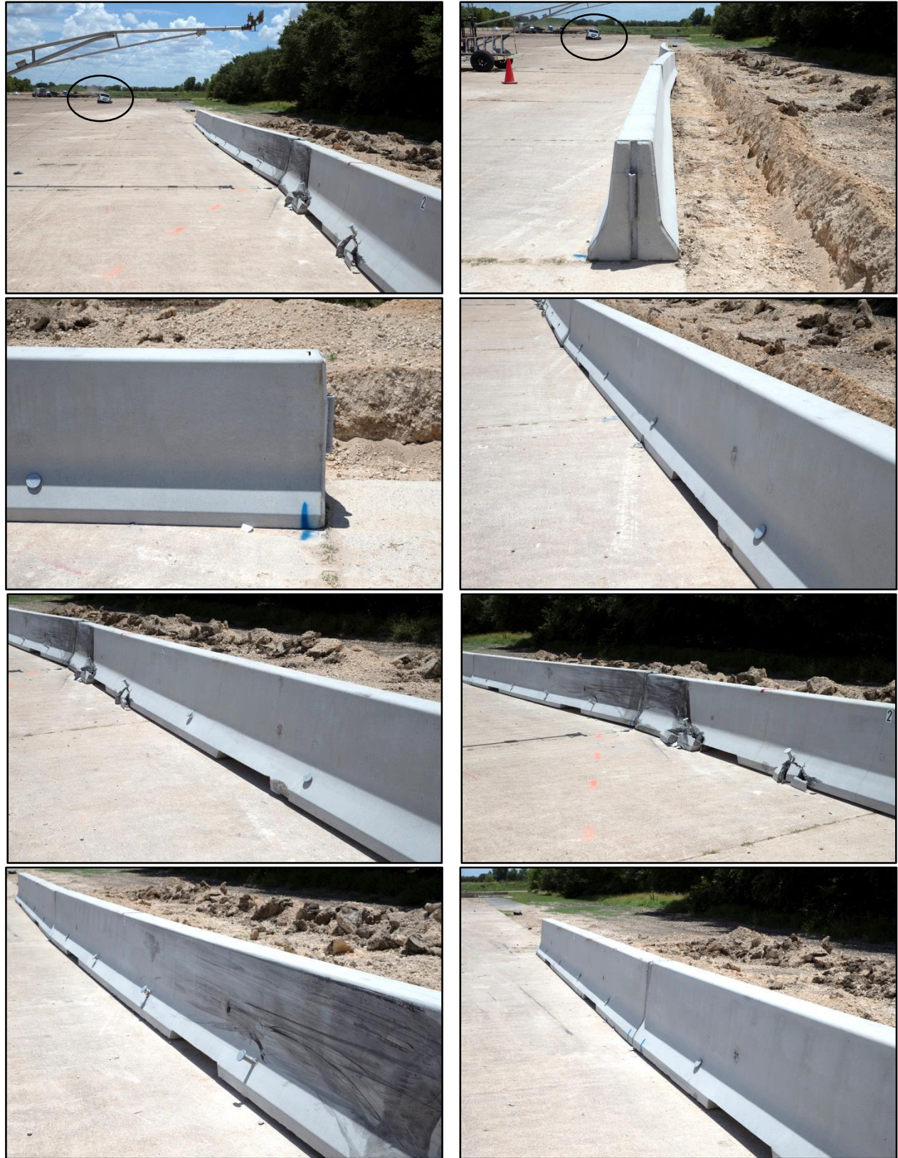
Figure 4.5. TxDOT 32-inch CSB(7)-10 Pinned to Concrete Pavement after Test No. 469467-5-1.
