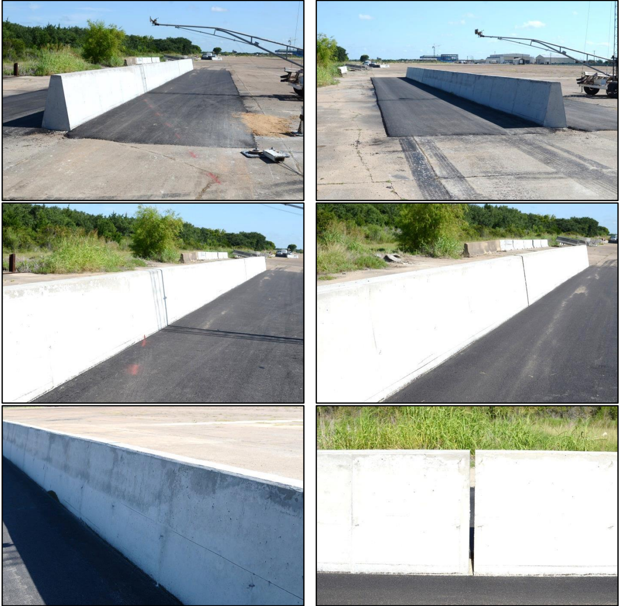
Figure 3.2. TxDOT 42-inch Tall SSCB with 1-inch ACP Overlay prior to Testing.
