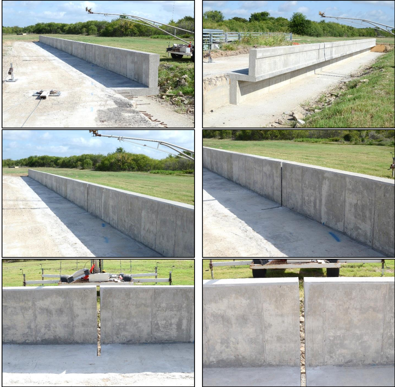
Figure 2.2. TxDOT 36-inch Vertical Concrete Bridge Rail prior to Testing.
