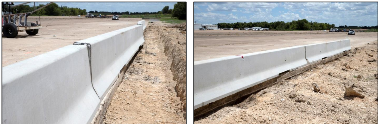
Figure 4.8. Field Side of Barrier after Test No. 469467-5-1.
