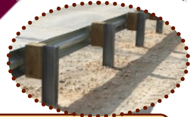
Strong-Post W-Beam Guardrail with 25" Height (TL-2)
