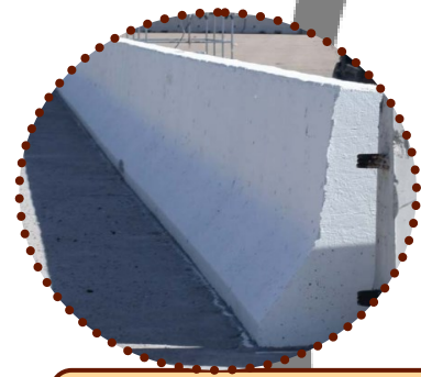
32" New Jersey Safety Shape Barrier (TL-3)
