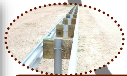
31" W-Beam Median Barrier (TL-3)
