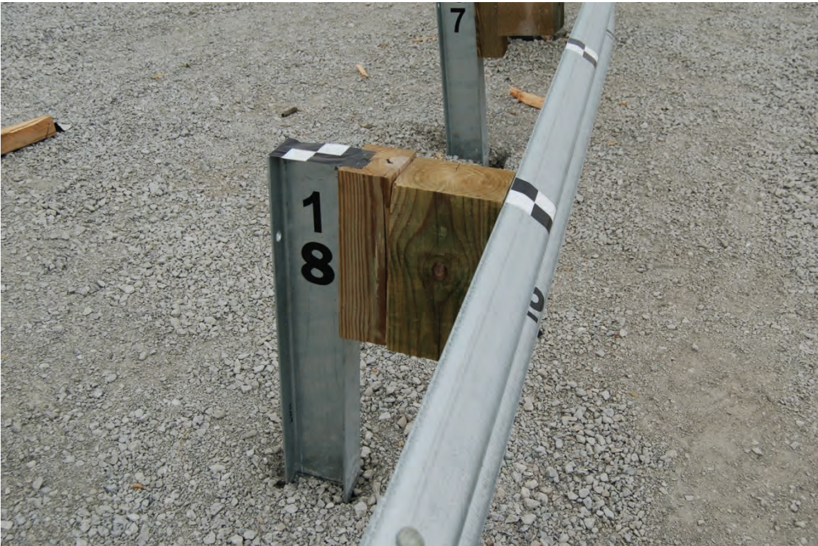
Figure 36. Post Nos. 17 and 18 Damage, Test No. MGSC-5
