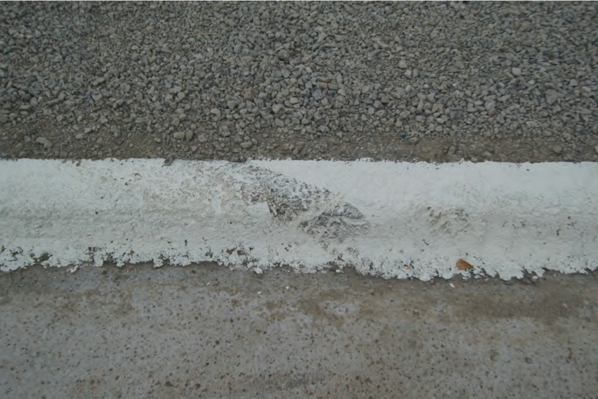
Figure 28. Curb Damage, Test No. MGSC-5
