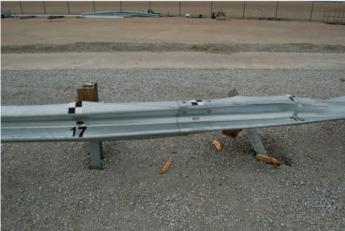
Figure 31. Rail Damage, Post Nos. 16 and 17, Test No. MGSC-5
