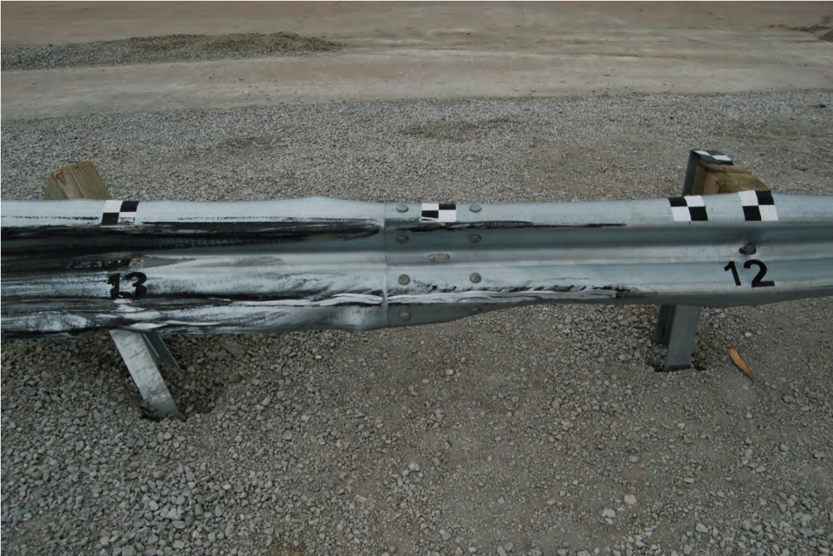
Figure 29. Rail Damage, Post Nos. 12 and 13, Test No. MGSC-5
