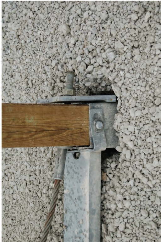
Figure 38. Upstream Anchorage Damage, Test No. MGSC-5
