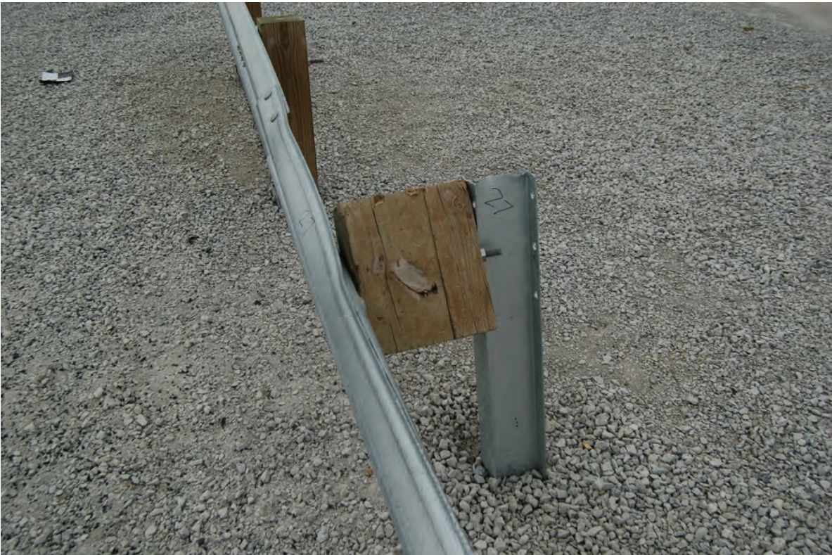
Figure 37. Post Nos. 26 and 27 Damage, Test No. MGSC-5
