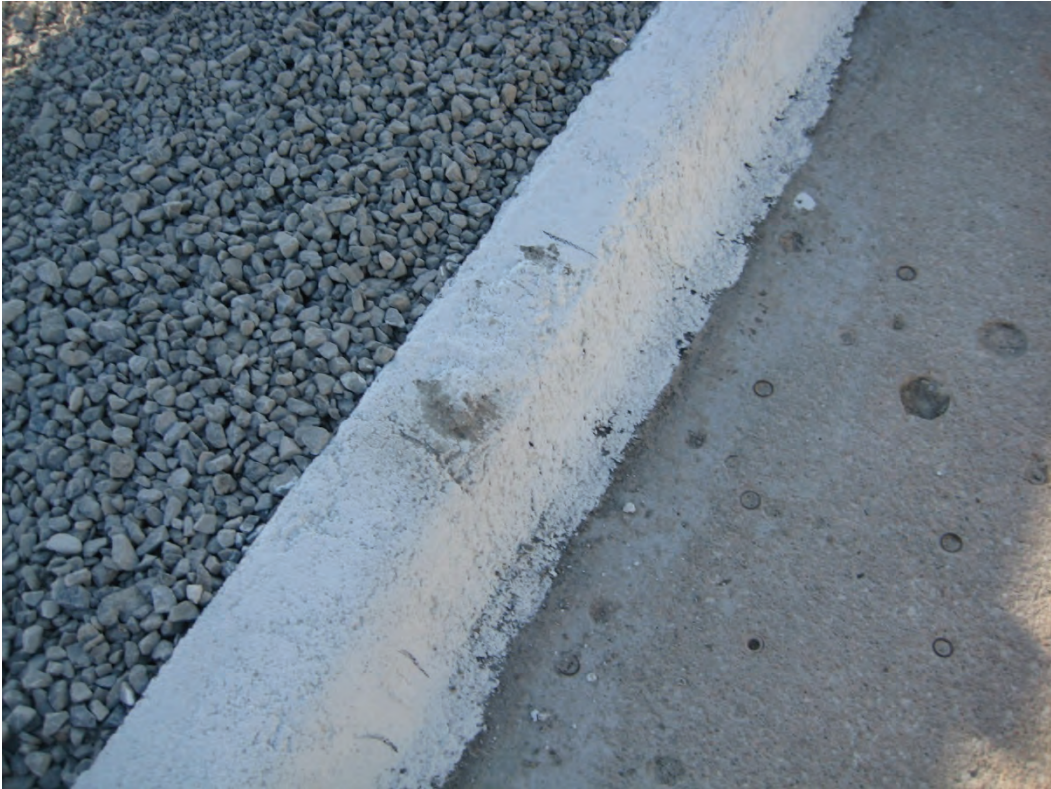
Figure 13. Test Installation Photographs, Test No. MGSC-5
