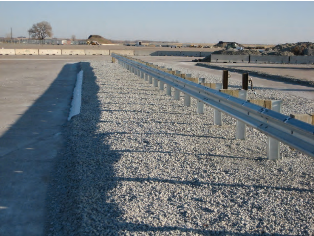
Figure 11. Test Installation Photographs, Test No. MGSC-5
