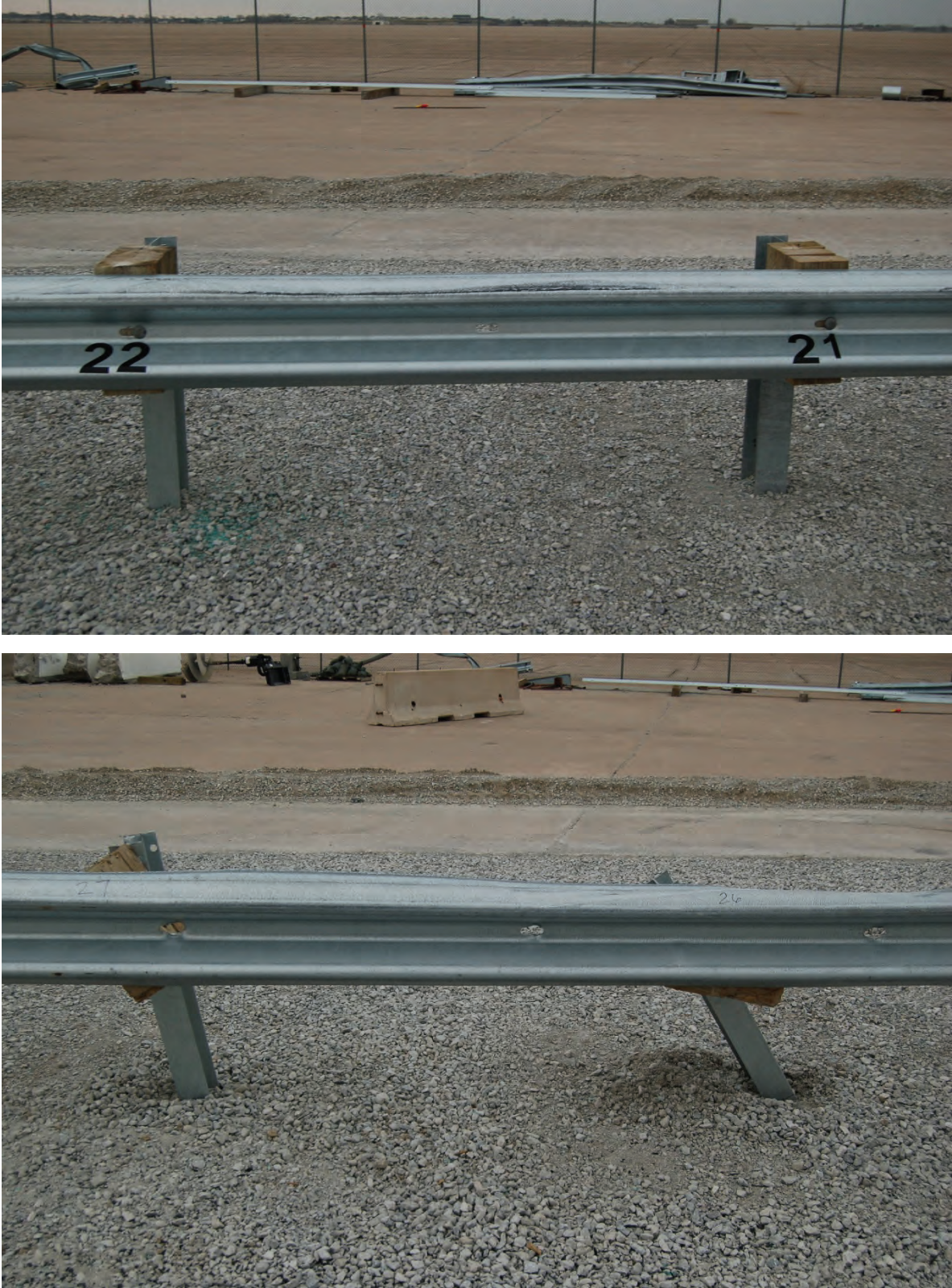
Figure 32. Rail Damage, Post Nos. 21, 22, 26, and 27, Test No. MGSC-5
