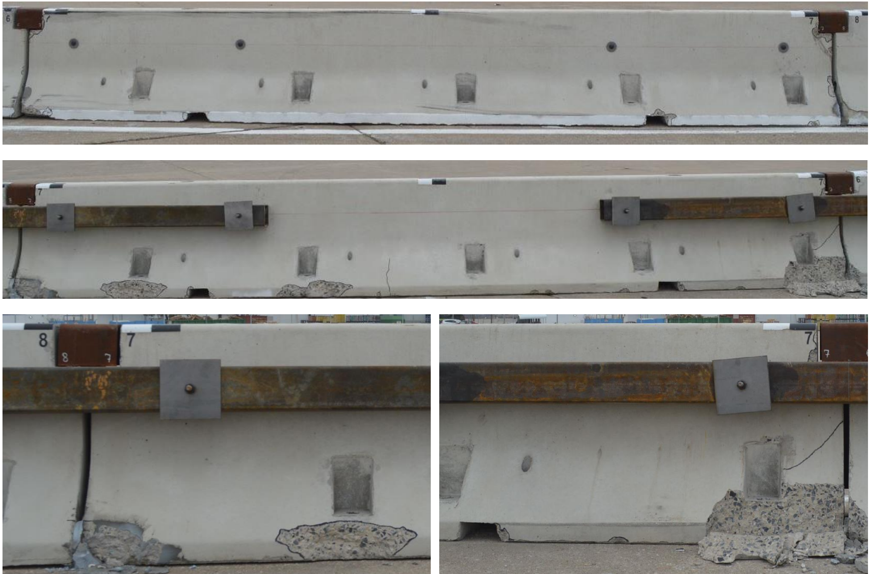
Figure 42. Barrier No. 7 – Traffic and Back Side Damage, Test No. NJPCB-5
