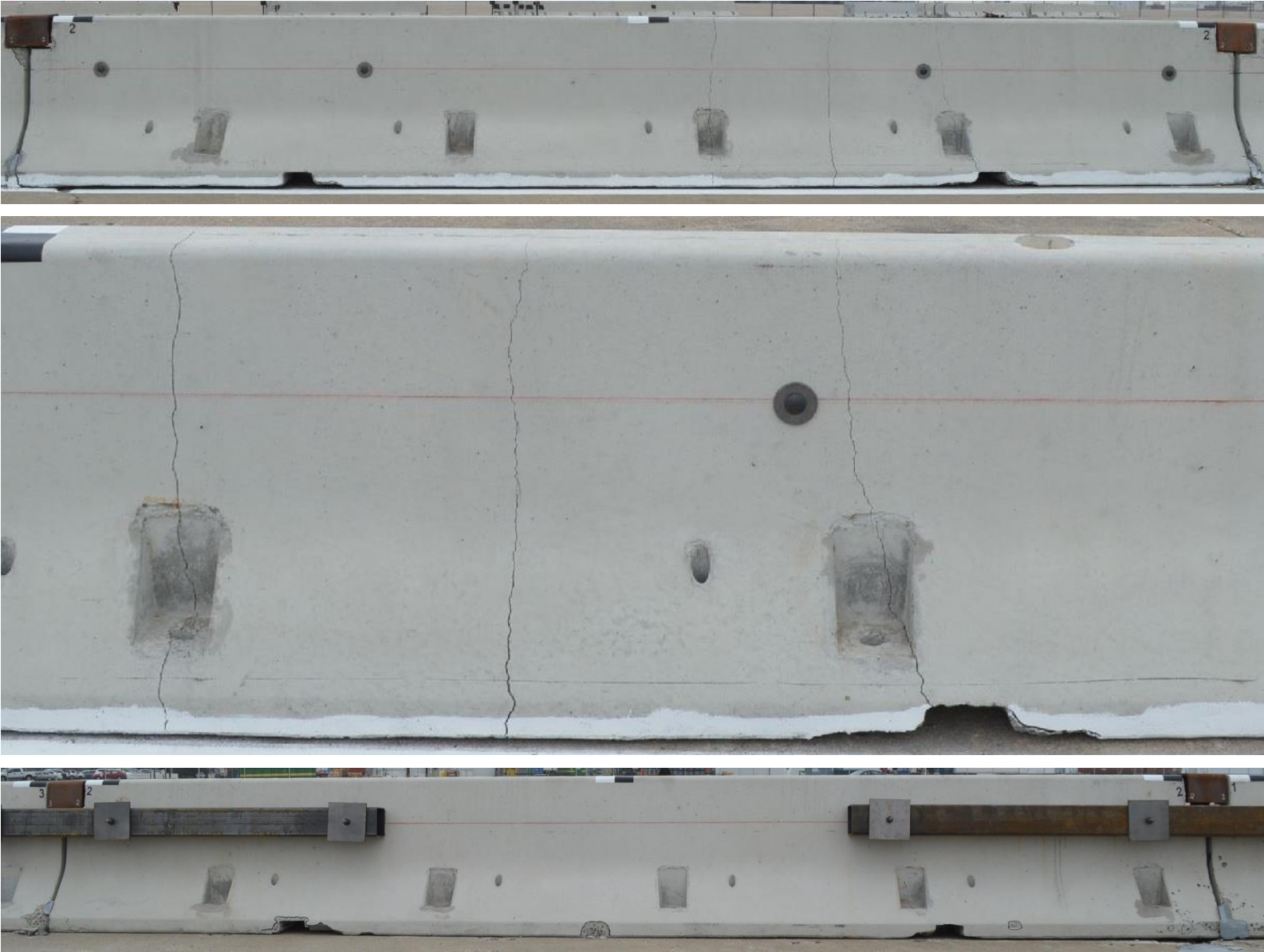
Figure 37. Barrier No. 2 – Traffic and Back Side Damage, Test No. NJPCB-5
