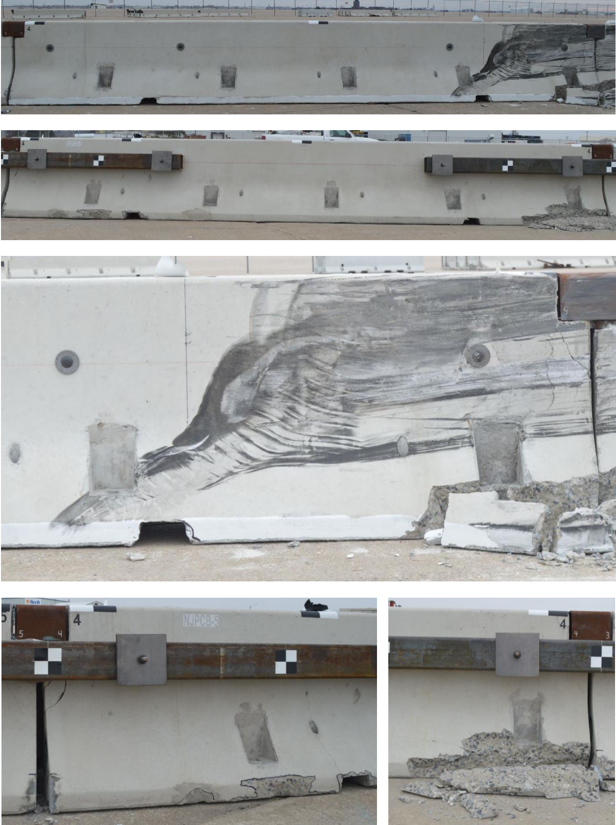
Figure 39. Barrier No. 4 – Traffic and Back Side Damage, Test No. NJPCB-5
