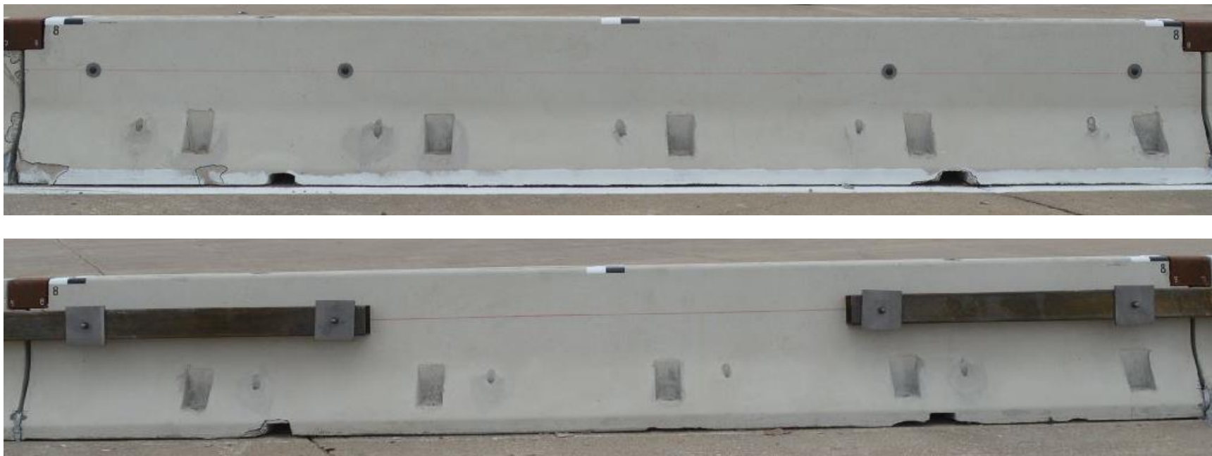
Figure 43. Barrier No. 8 – Traffic and Back Side Damage, Test No. NJPCB-5
