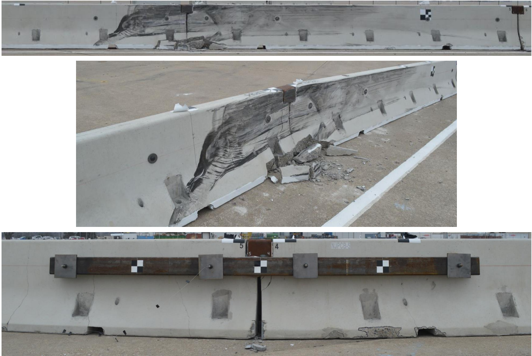
Figure 36. System Damage at Impact Location, Front and Back Side, Test No. NJPCB-5
