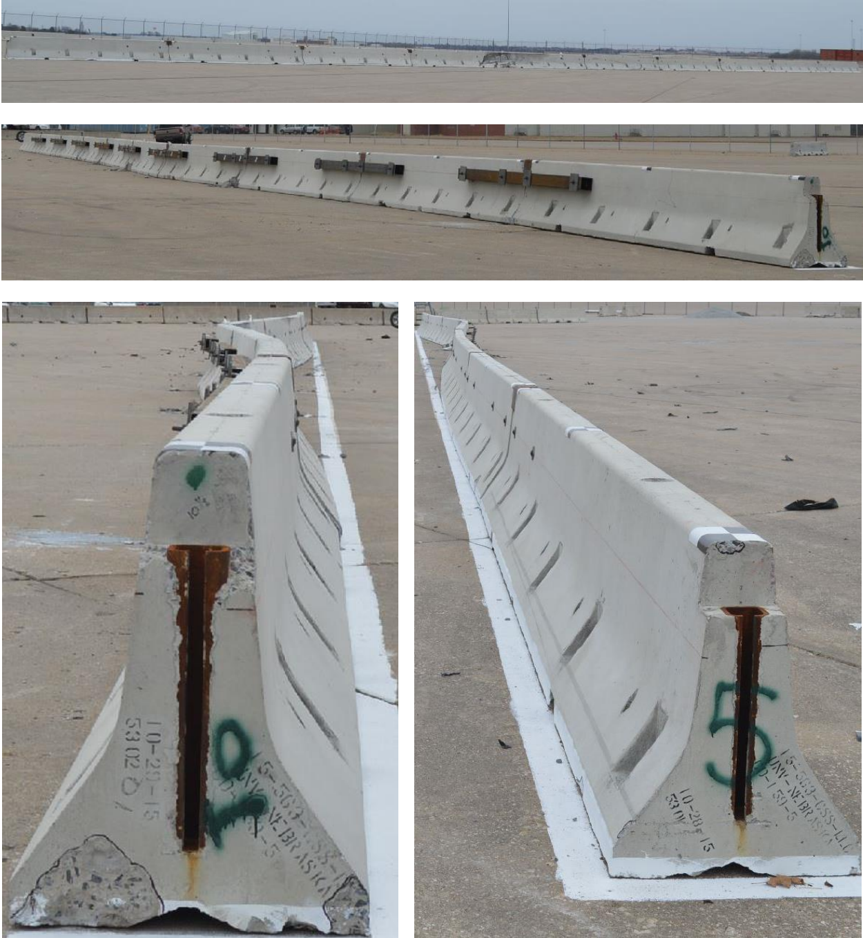
Figure 35. System Damage - Front, Back, Upstream, and Downstream Views, Test No. NJPCB-5
