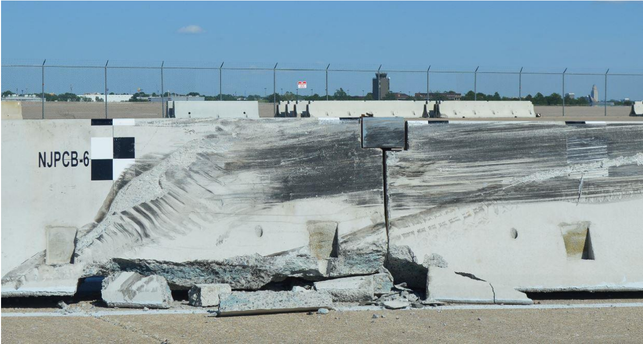
Figure 36. Barrier Nos. 4 and 5 Damage, Test No. NJPCB-6
