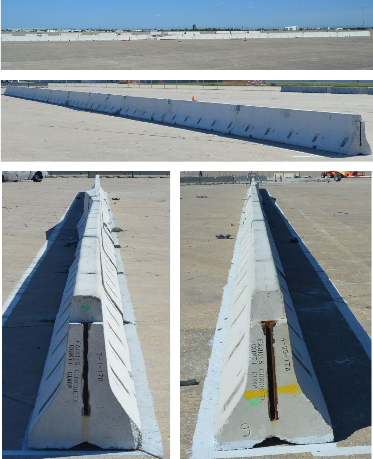
Figure 34. System Damage – Front, Back, Upstream and Downstream Views, Test No. NJPCB-6
