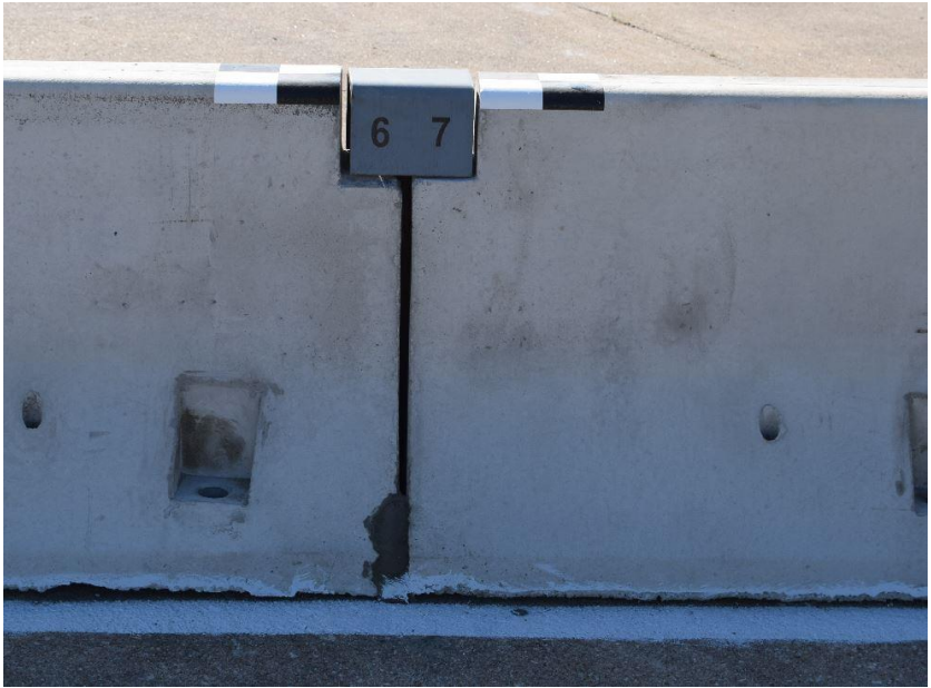
Figure 16. PCB Connection Key and Connection Socket, Test No. NJPCB-6
