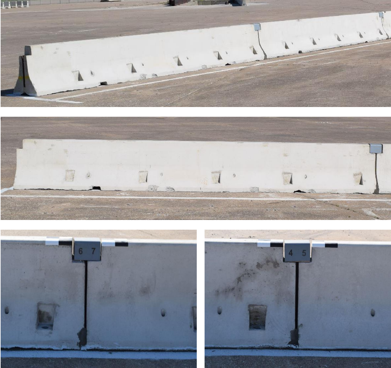
Figure 18. Grout at Toes Between PCBs, Test No. NJPCB-6
