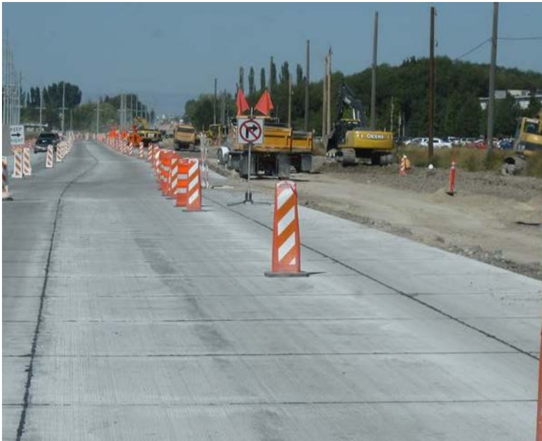
Figure 2. Proper sign height among channelizing devices.
