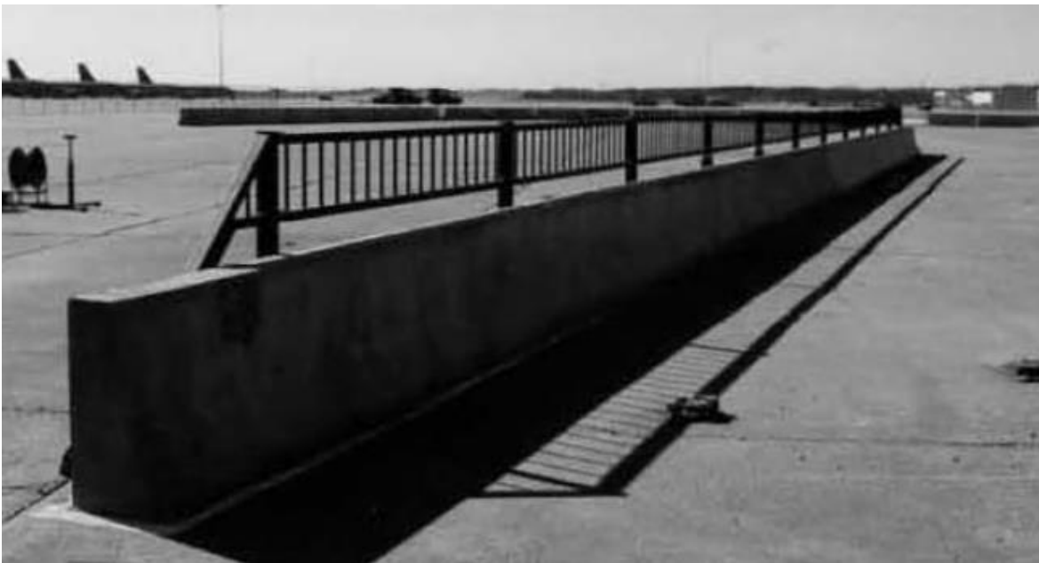
Figure 8. Minnesota Combination Traffic/Bicycle Rail [14]
