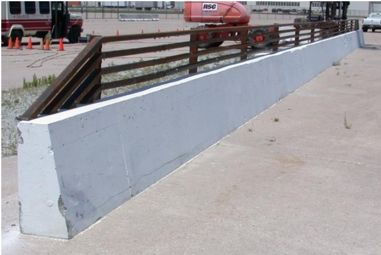
Figure 9. Missouri Combination Rail with Four Rail Elements [15]
