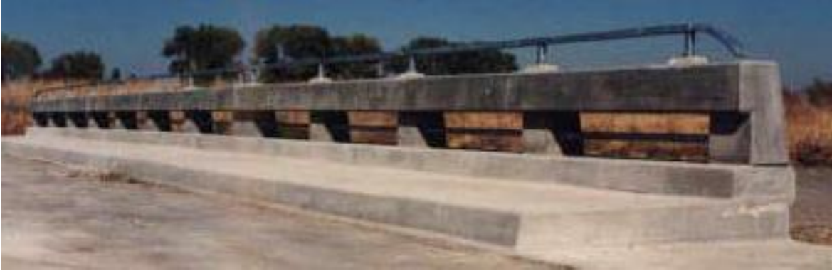
Figure 7. Type 80 SW Bridge Railing [13]
