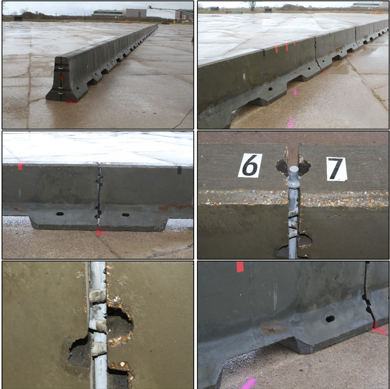
Figure 5.2. Free-Standing F-Shape Barrier with Drainage Scuppers Prior to Testing.
