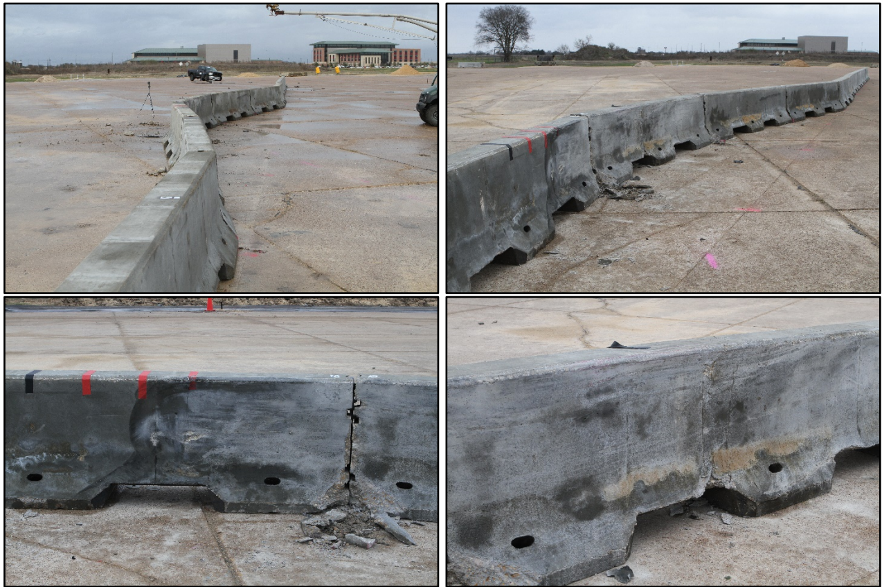
Figure 5.5. Barrier after Test No. 612831-01-2.
