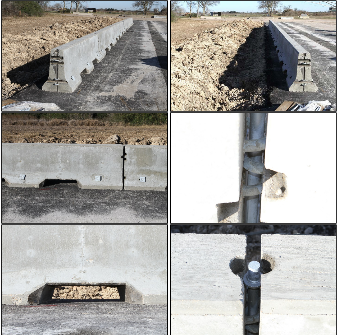
Figure 4.2. Pinned F-Shape Barrier with Drainage Scuppers prior to Testing.
