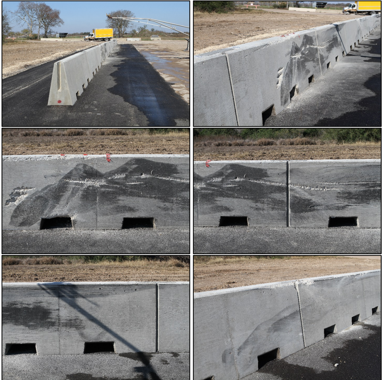
Figure 6.5. Embedded Single-Slope Barrier with Scuppers after Test No. 612831-01-3.
