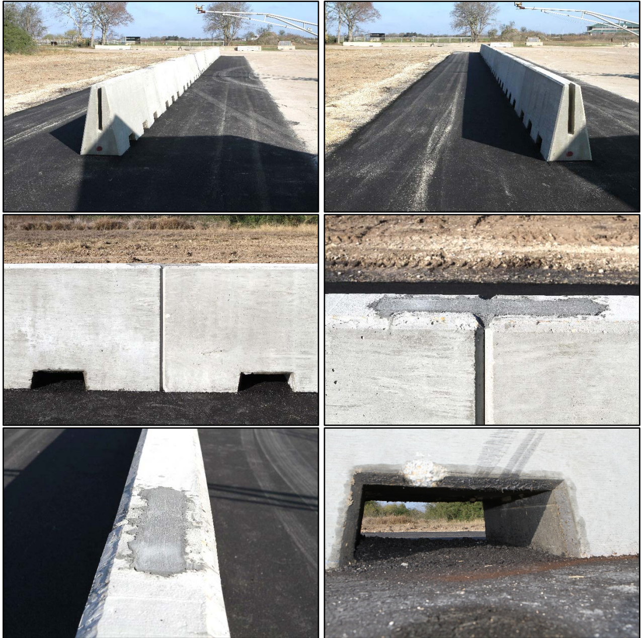
Figure 6.2. Embedded Single-Slope Barrier with Drainage Scuppers Prior to Testing.
