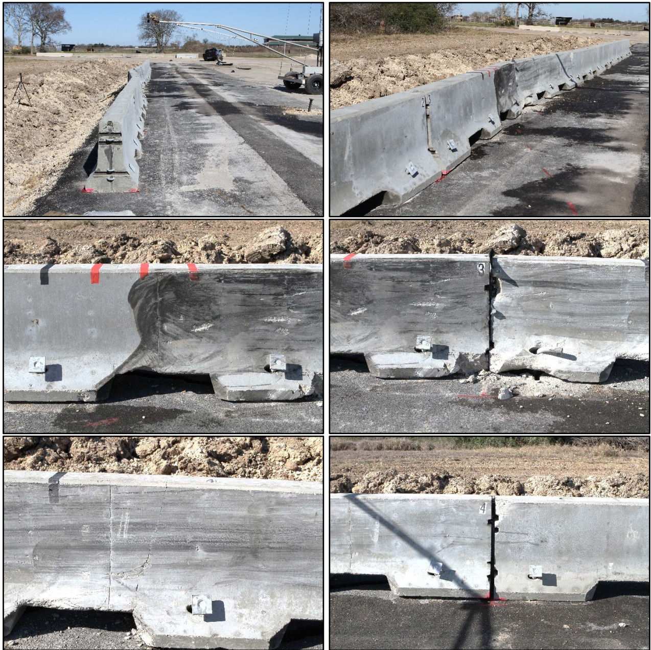
Figure 4.5. Barrier after Test No. 612831-01-1.
