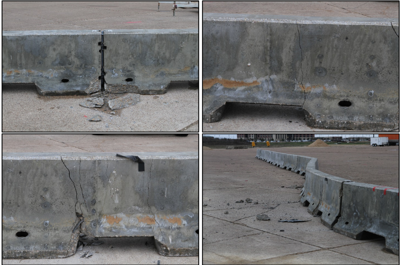
Figure 5.6. Field Side of Barrier after Test No. 612831-01-2.
